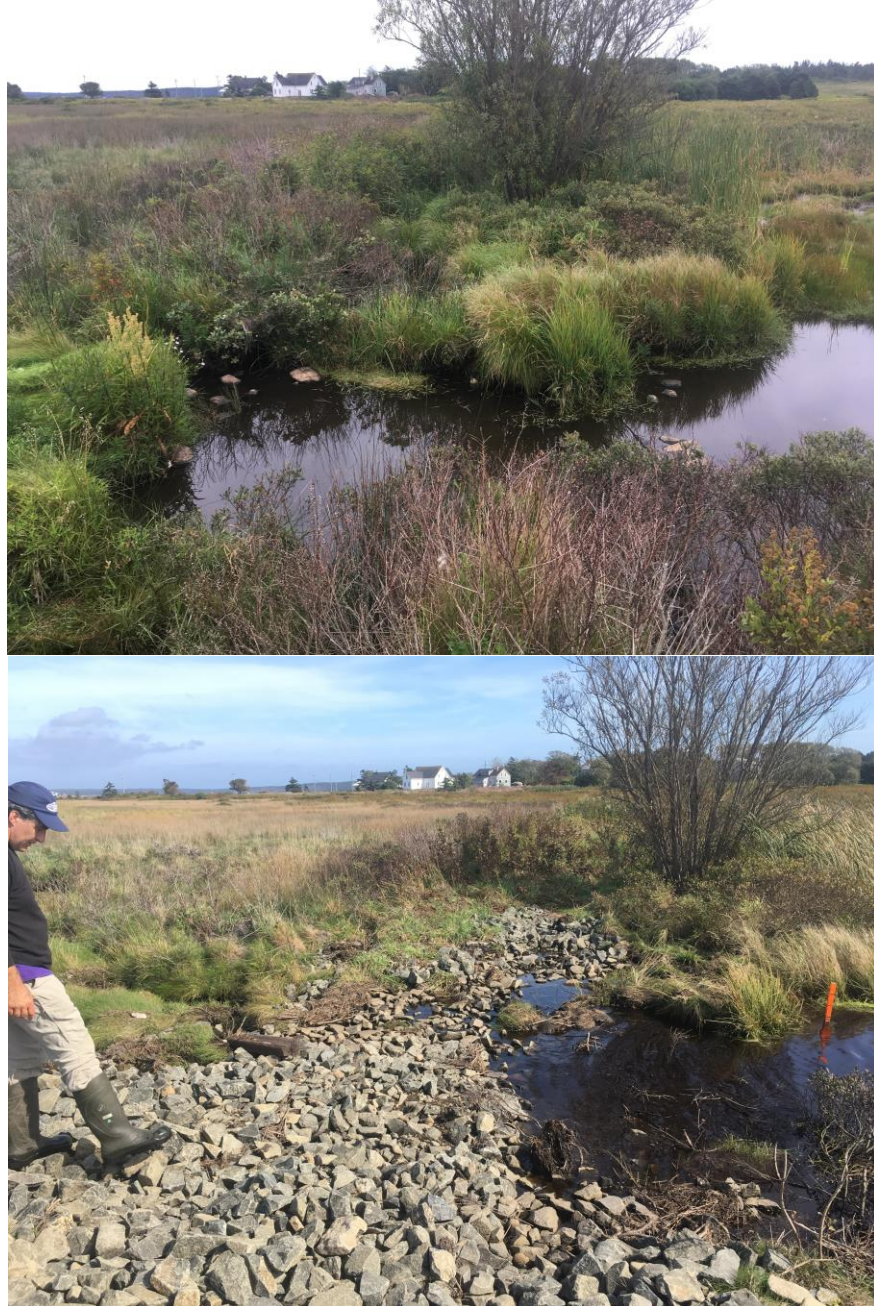
Figure 29: Pre and post restoration views of Jimmy's pond outlet channel. The outlet was raised .03-0.4 m and armoured for stability.
