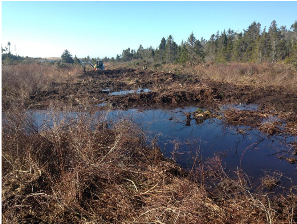
Figure 10: Following significant rain during initial construction, ditchblocks immediately impounded water and redirected sheet flows to the reactivated lagg channel rather than along the ditch.
