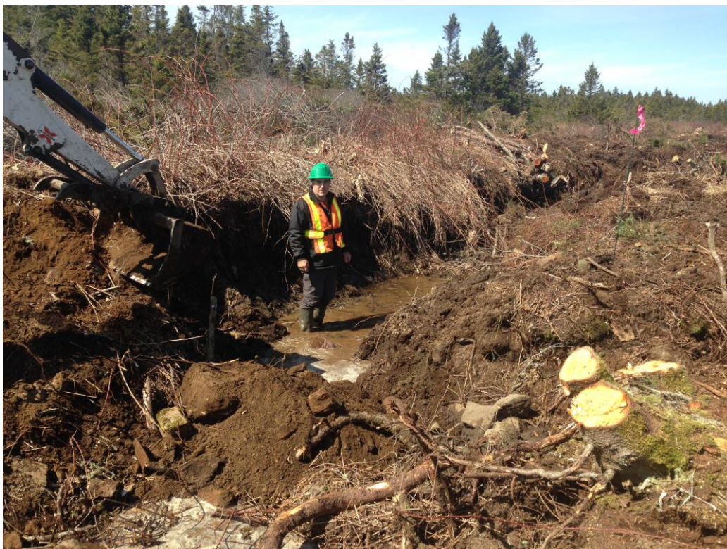
Figure 8: The mineral, rather than peat, nature of soils near big Pond are visible in this image, as is the relative depth of the Southwest ditch prior to remediation.
