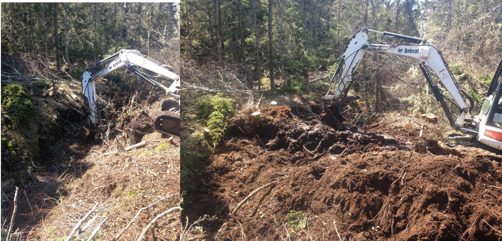
Figure 20: A before (L) and after (R) of ditchblock construction on the southeast ditch in a heavily forested stretch. Note that ditch has become dry from construction of upslope ditchblocks, allowing work to occur “in the dry”. In the nearly completed photo (R), the ditchblock of wet catotelmic peat under the excavator buck is being compacted with an initial sod being placed on top of the far end of the ditchblock. Note the dry desiccated shallow peat piled in the image foreground that has been removed to allow access to deeper wet peat used in construction.
