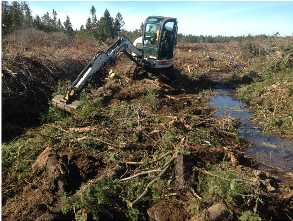
Figure 9: The natural lagg channel (photo right) was reactivated with stream flow following the initial upslope ditchblock installation, allowing the remaining ditch work (photo left) to be carried out "in the dry".
