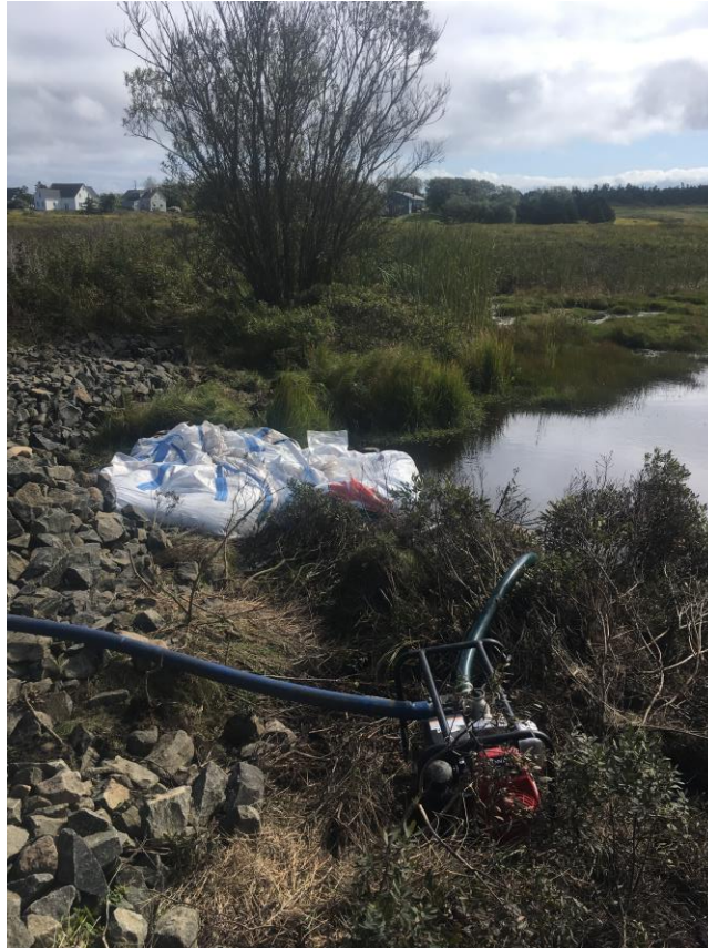
Figure 25: Cofferdam bags isolate the outflow from Jimmy's Pond, while a 2" pump was used to draw down the pond water level prior to restoration works.
