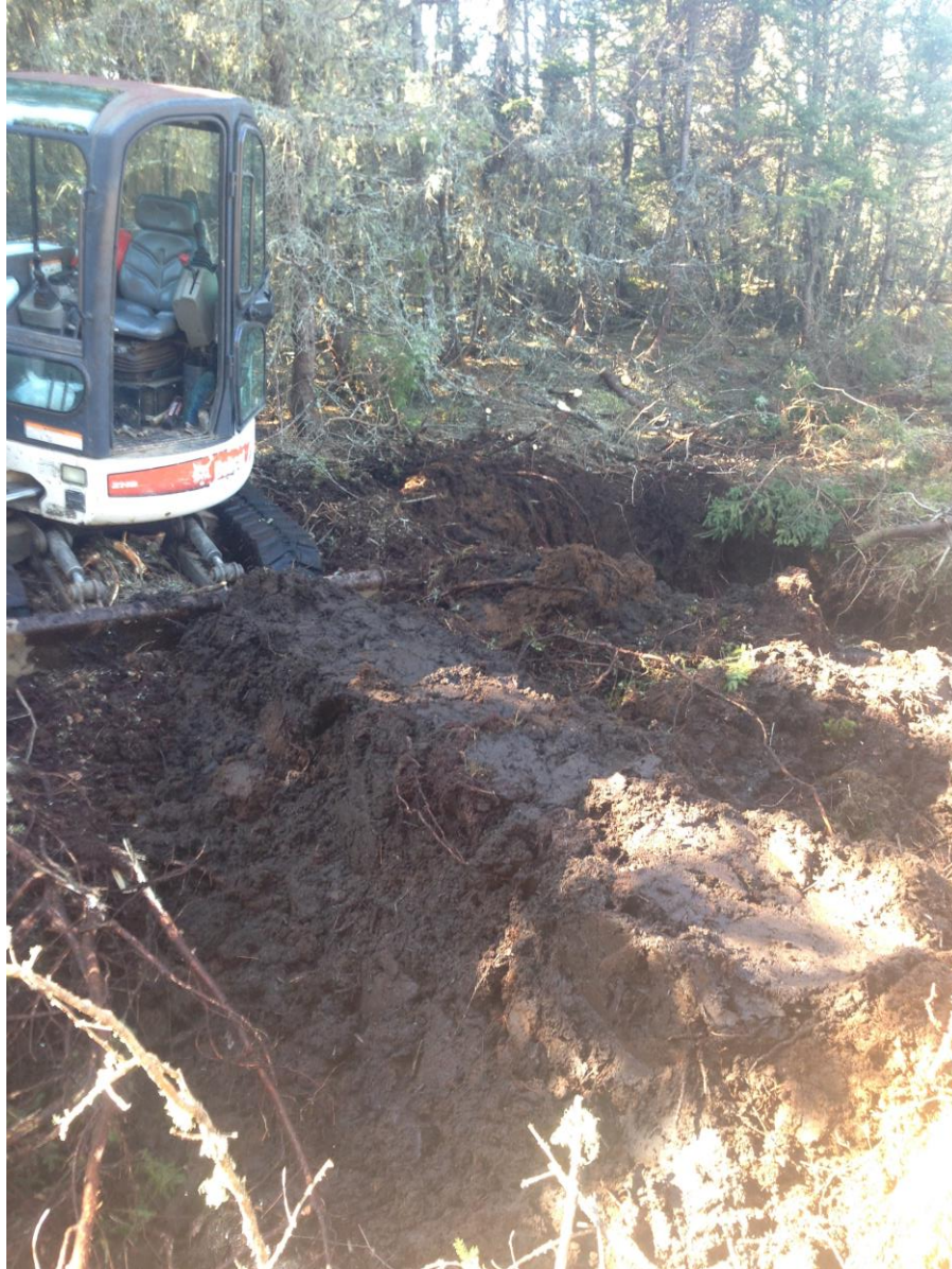
Figure 19: A ditchblock nears completion on the southeast ditch. The compacted peat core is visible, waiting to be topped with available live "sod" that will promote quick growth and stability.
