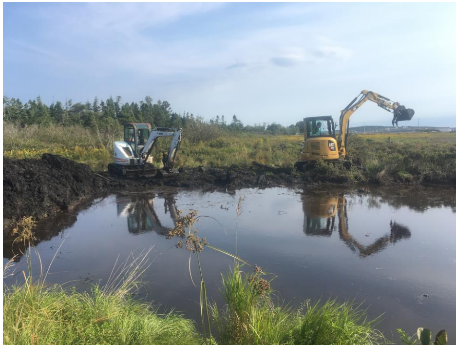
Figure 26: Compact excavators sit on timber cribbing to excavate the pond infill.
