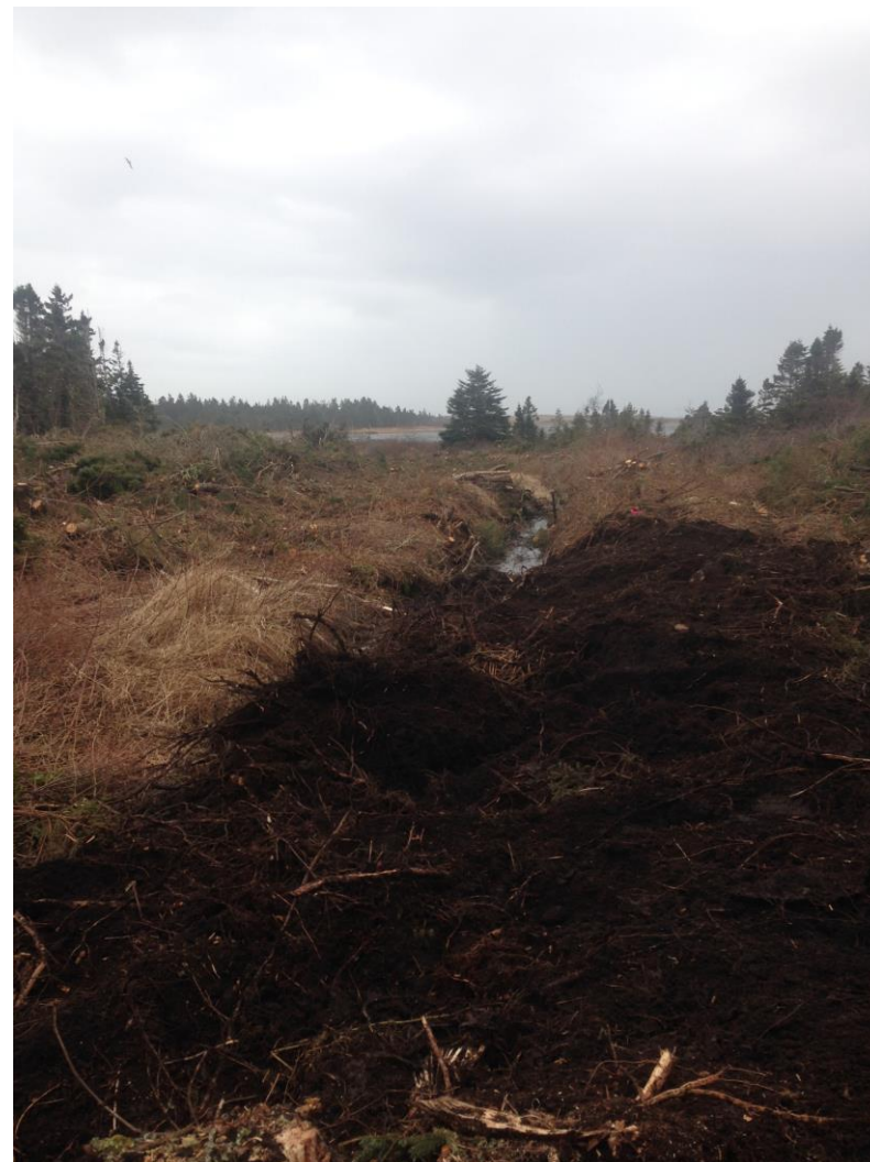
Figure 11: A view south along the southwest ditch toward Big Pond following tree cutting, and during clearing of the construction corridor along the brook (L) and following initial re-profiling activities (R).
