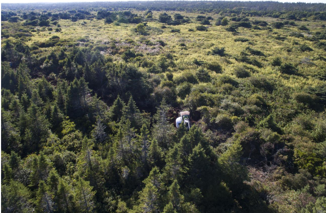
Figure 17: An excavator works in a recently cut corridor of trees along the north east ditch. The view is south westward across Big Meadow Bog and shows the scattered encroachment of larger trees across the main bog that would be felled as a final step in the restoration process. (Photo credit: Mike Dembeck photography mikedembeck.com )
