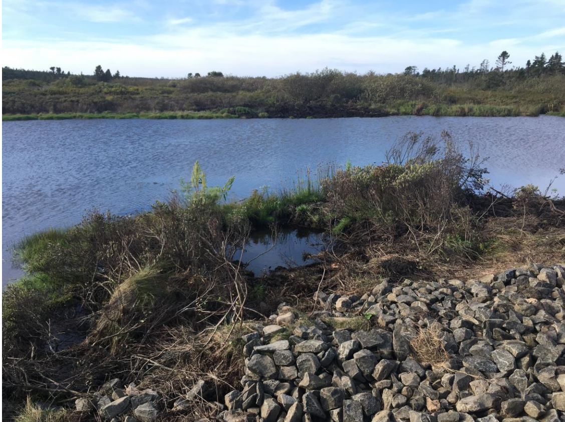
Figure 28: Distant trees provide reference for this pre (Aug 2017) and post (Sept 2017) restoration southward view of the pond toward Big Meadow Bog. Stone in the foreground is part of the restored outlet channel, which further raised the water level within the pond.
