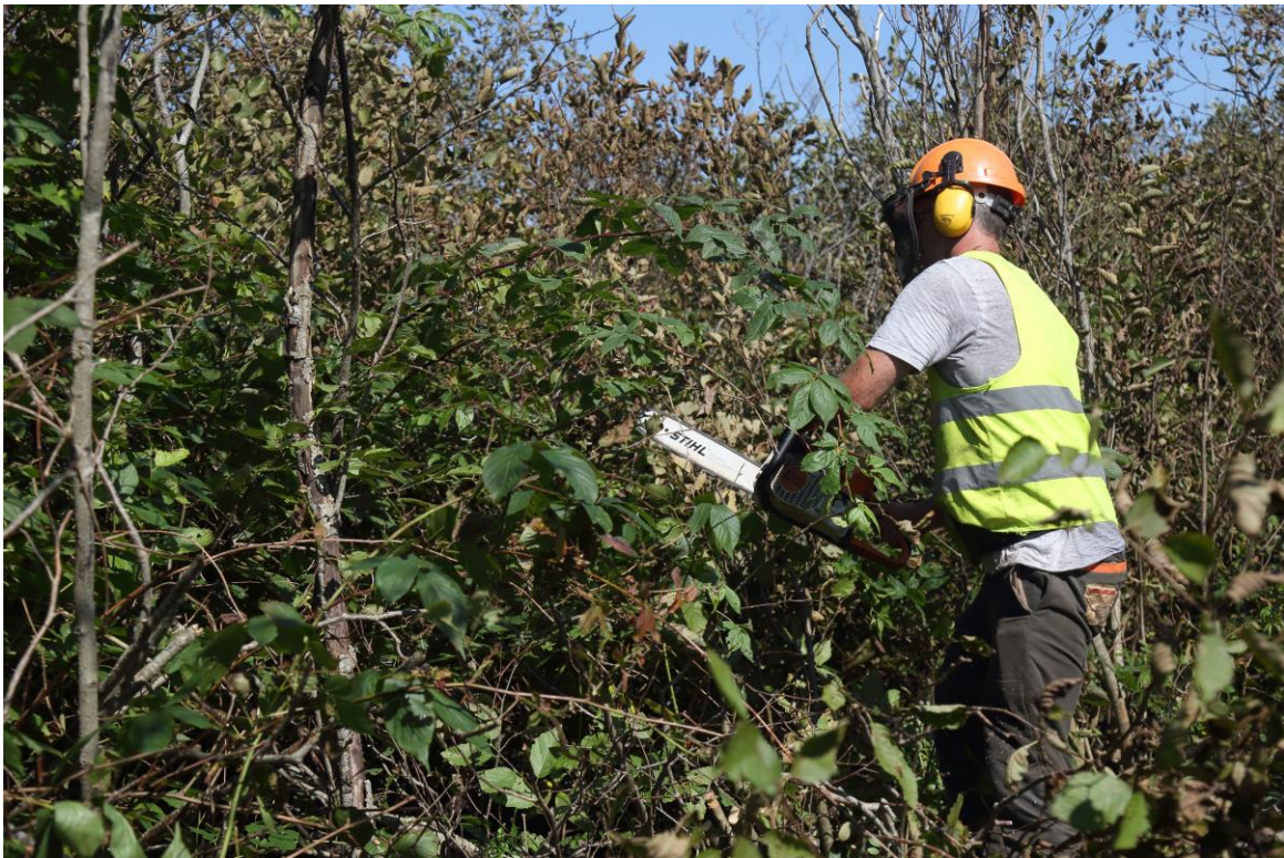
Figure 14: Dense tree/tall shrub growth along historic ditch lines had to be cut prior to restoration to gain machine access. Here, an alder stand in the north confluence is cleared.
