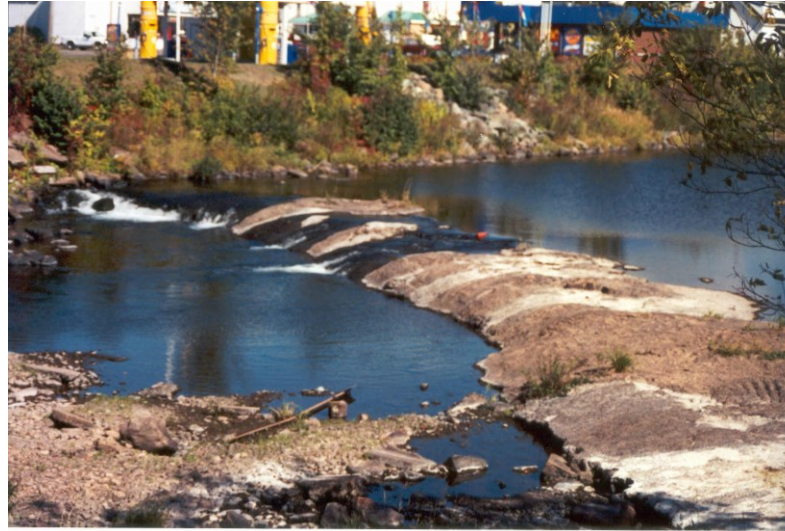
Photo 4: A cement cap helps protect a pipeline crossing of the Salmon River at Truro. At low flows, such as in the photo, it could inhibit some fish passage.
