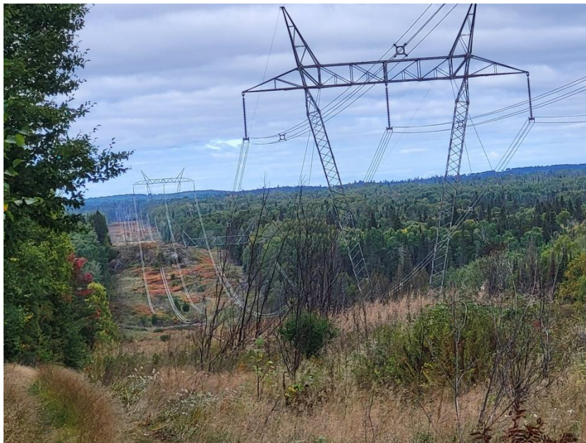
Figure 8 Photo of the hydro lines to the west of the property.
