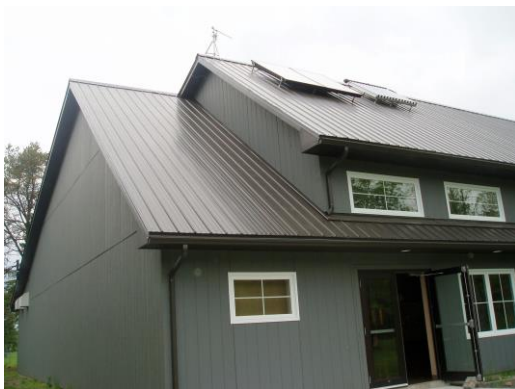
Roof-mounted solar water heaters: Flat-plate on left Evacuated tube on right
