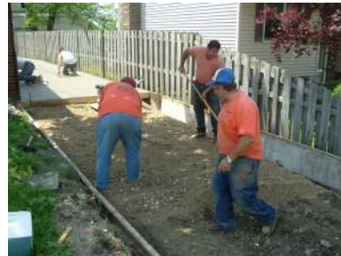
Installation of Formwork For New UFAS Compliant Pathway
