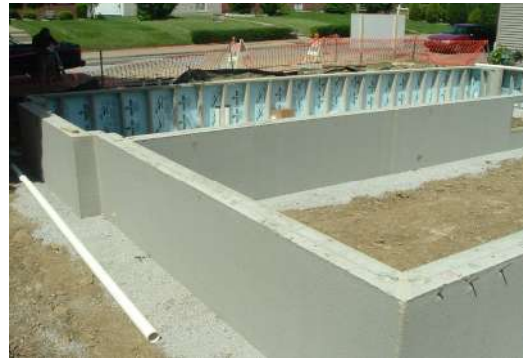
Foundation For a UFAS Compliant Two Bedroom Unit
