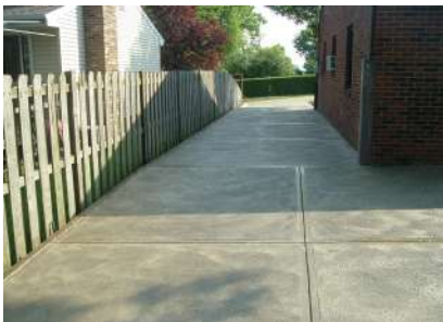
Recently Constructed UFAS Compliant Pathway
