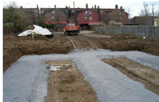
Foundation Pad For a UFAS Compliant Three Bedroom Unit
