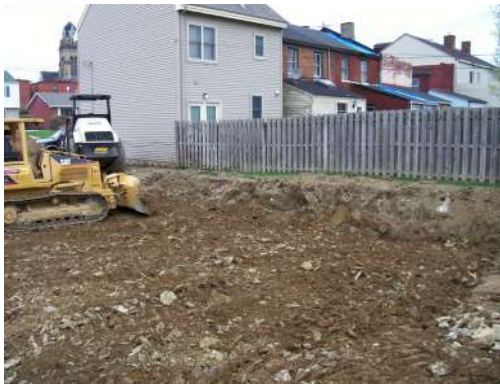
Site Preparation for a UFAS Structure
