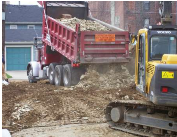
Site Grading for a UFAS Structure
