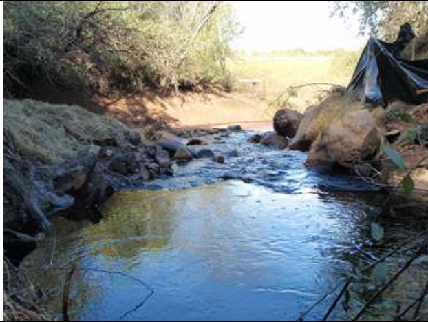
Water level downstream view of new channel, low tide
