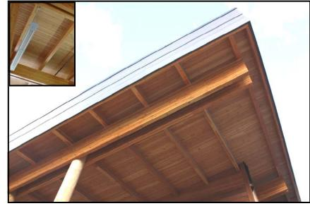
Enman Lumber were; the 2 x 6 Select Tight Knot, Fir Decking used for the interior and exterior ceilings. This product has been utilized frequently where appearance and load bearing features are important. In addition, various Western Red
