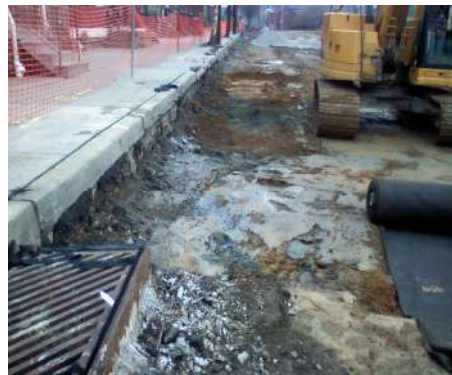
Overexcavation of Unsuitable Material
