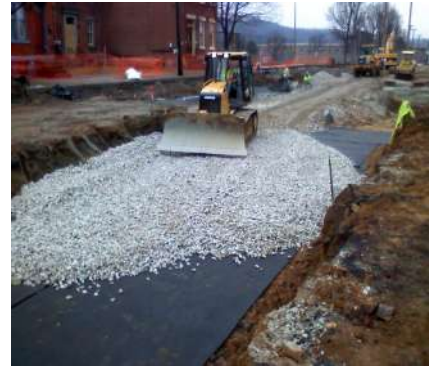
Installation of Foundation Mat and Base Course
