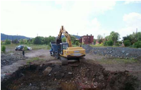
Site Preparation Activities UFAS Compliant Modular Housing Units
