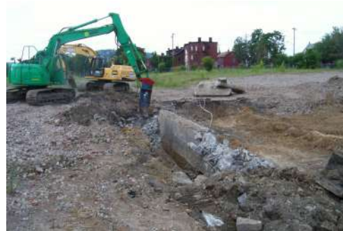
Site Preparation Activities UFAS Compliant Modular Housing Units
