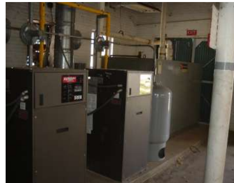
Power Control and Distribution
