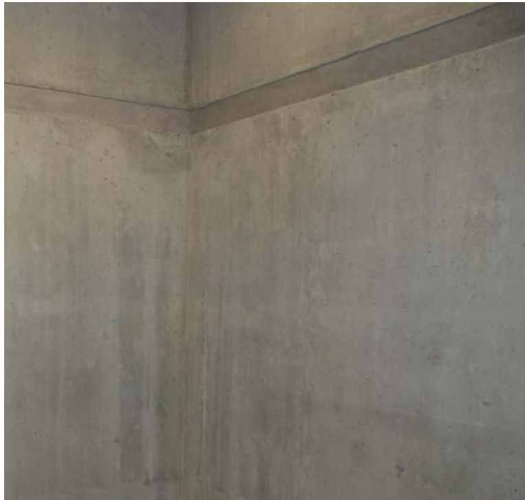
Figure 1 – Concrete Finish CF-1, Smooth Form Finish: Smooth formed surfaces free from bug holes larger than 4 mm, with no honeycombing, staining and paste wash down from subsequent concrete pours for multi-staged placement; and having evenly spaced form tie holes.
