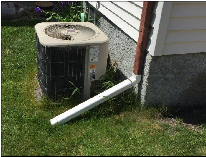
2. Downspouts end too close to building
