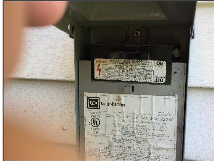
17. A/C electrical disconnect present
