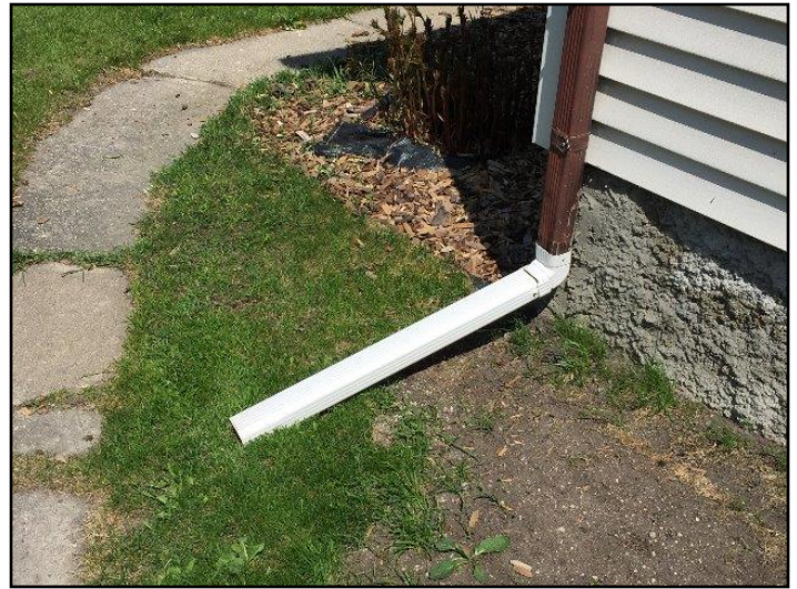
3. Downspouts end too close to building
