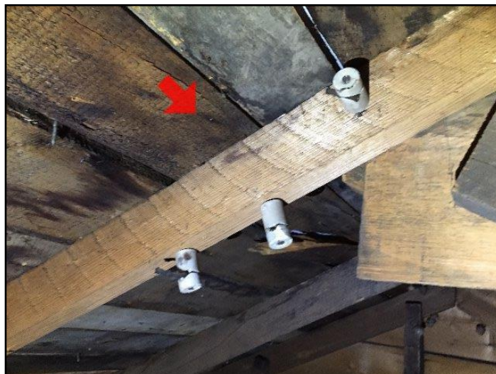
11. Copper - knob and tube
