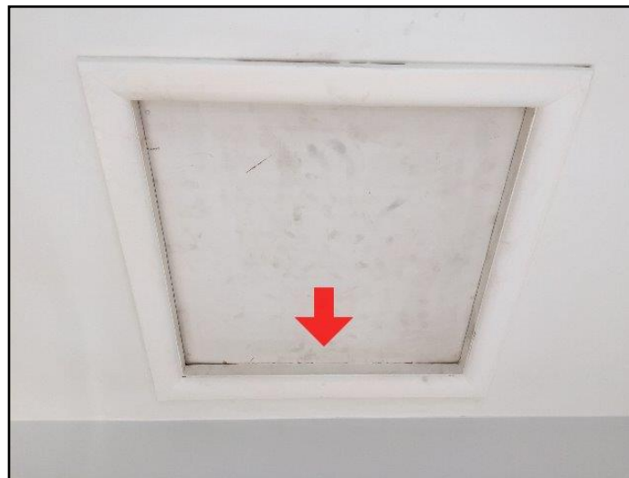
22. Not insulated and not weatherstripped
