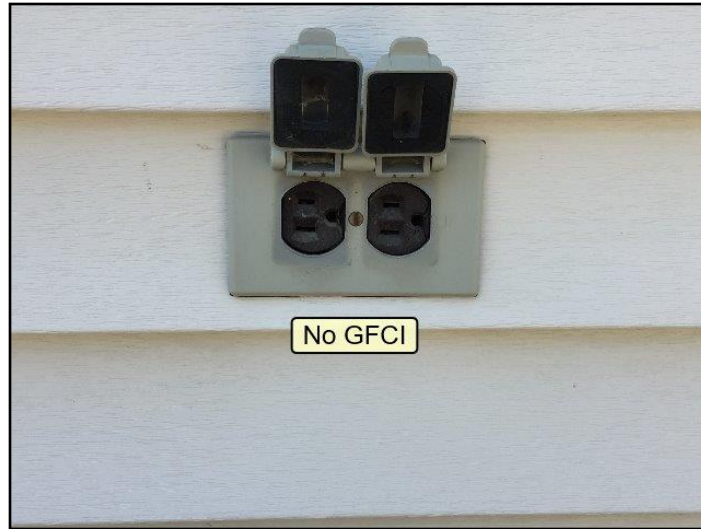
14. No GFCI/GFI (Ground Fault Circuit...
