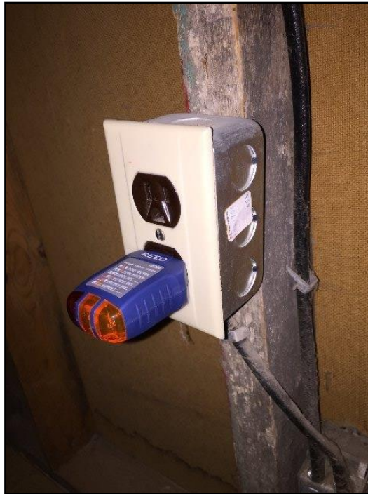
13. Ground needed for 3-slot outlet
