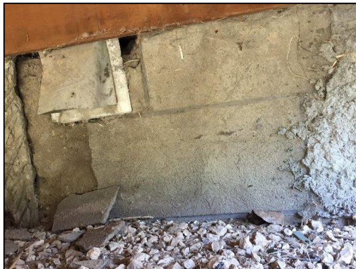
7. Parging damaged or missing
