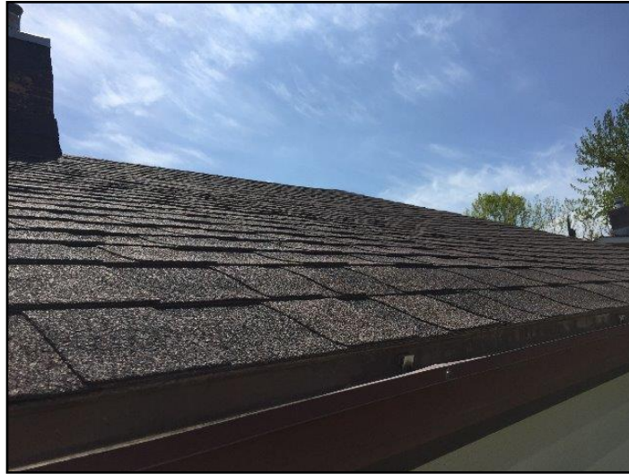
1. Asphalt shingles
