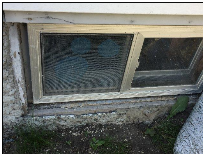
4. Caulking loose, missing or deteriorated
