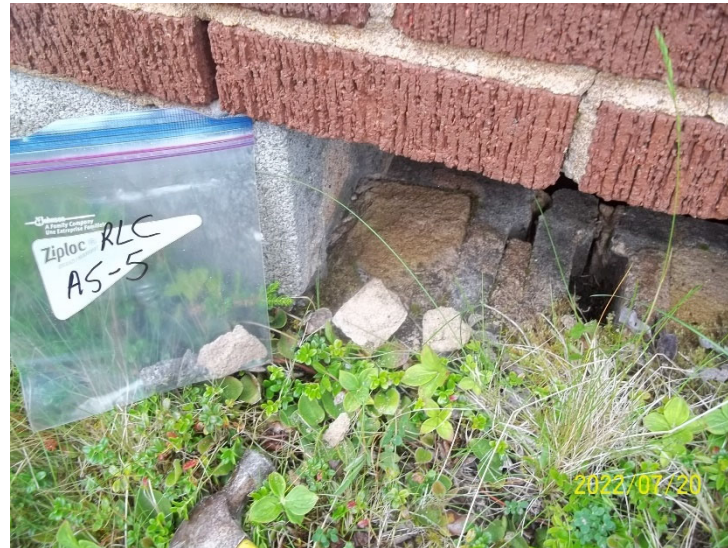
Photo 12: View of bulk material sample RLC AS-5, cinder block and mortar, cabin exterior.
