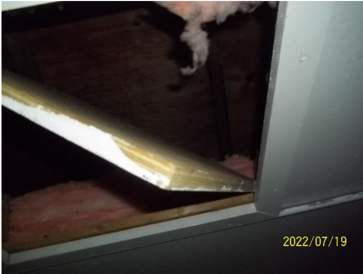
Photo 9: View of the attic in the accommodations cabin at Camp 50.
