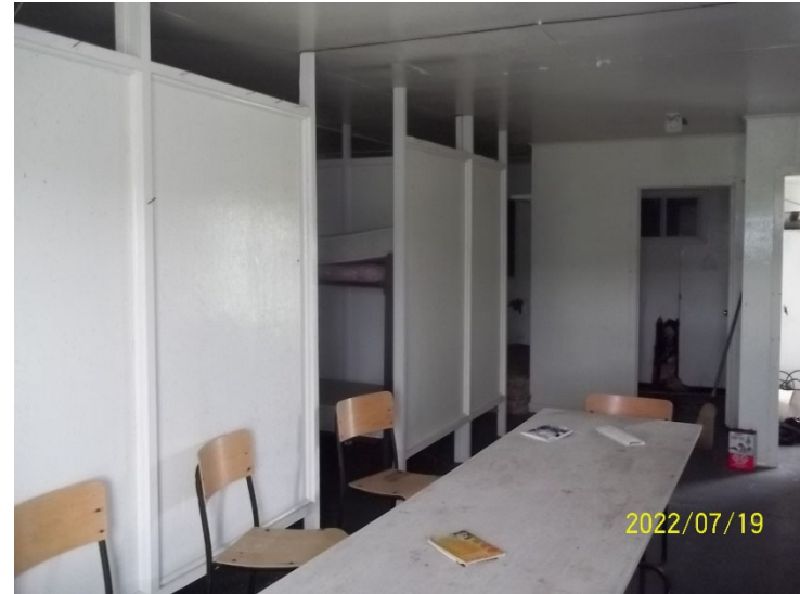
Photo 6: View of the dining area of the accommodations cabin at Camp 98.
