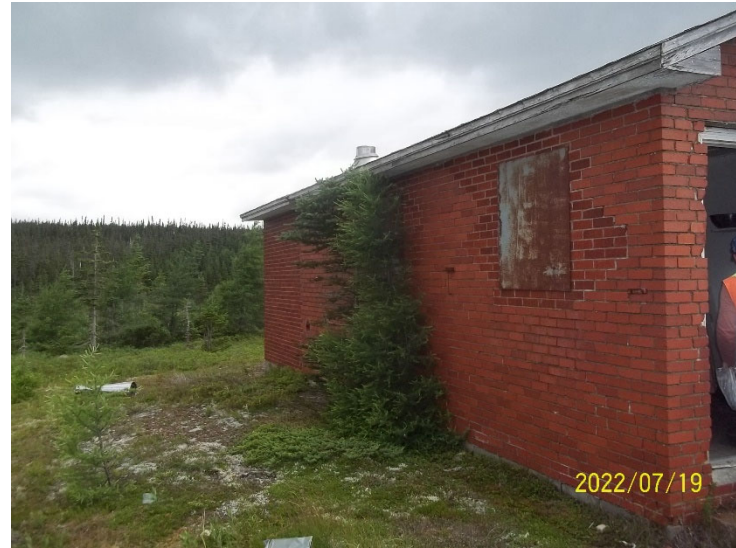
Photo 2: View of the accommodations cabin at Camp 98.
