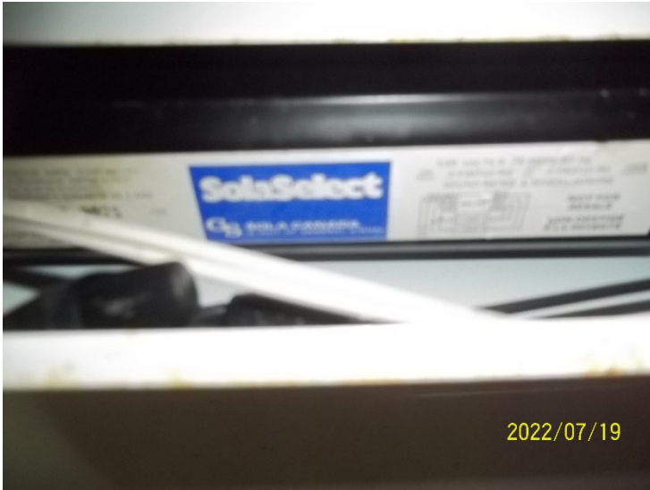
Photo 25: View of fluorescent light ballast inside the accomodations cabin.
