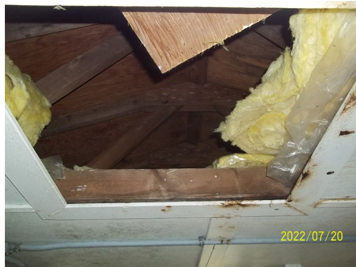
Photo 10: View of the attic inside the accommodations cabin at Glover Island Camp.
