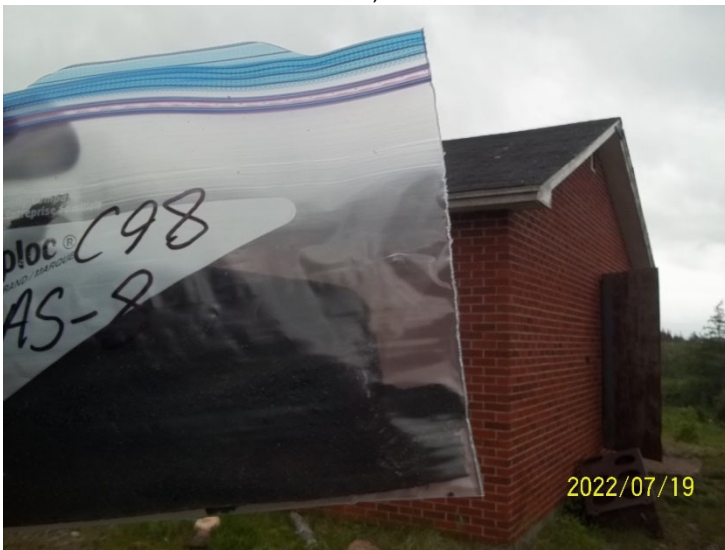
Photo 19: View of bulk material sample C98 AS-8, shingle, cabin exterior.
