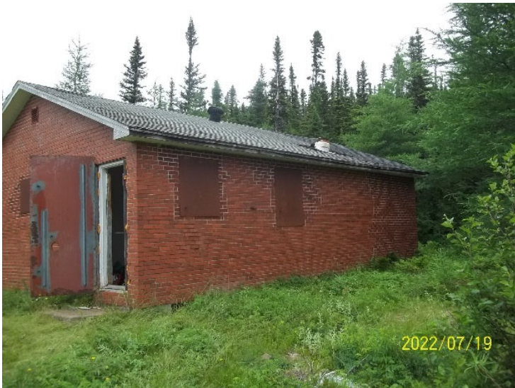
Photo 3: View of the accommodations cabin at Camp 50 site.
