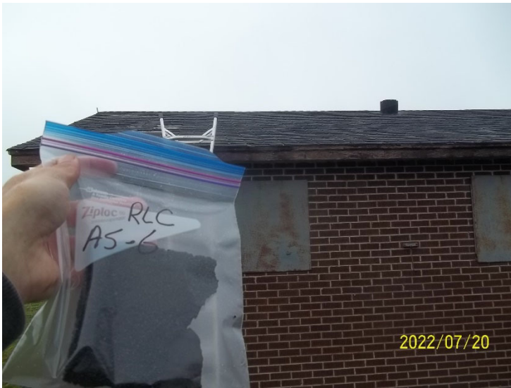
Photo 13: View of bulk material sample RLC AS-6, shingle, cabin exterior.
