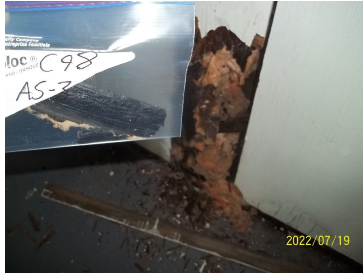
Photo 14: View of bulk material sample C98 AS-3, tar paper, cabin interior.
