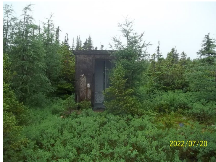
Photo 12: View of the outhouse at Rainy Lake Camp.
