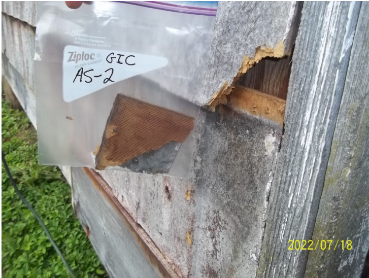
Photo 13: View of bulk material sample GIC AS-2, particle board, cabin exterior.
