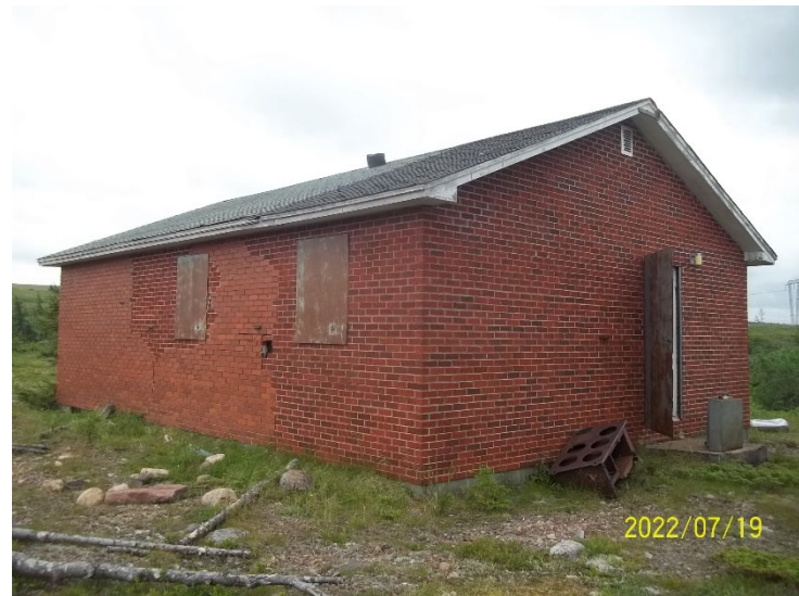
Photo 4: View of the accommodations cabin at Camp 98.
