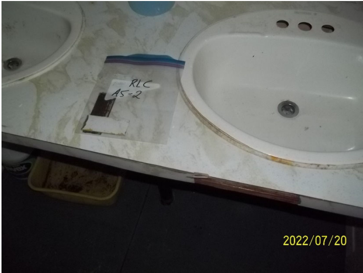
Photo 9: View of bulk material sample RLC AS-2, countertop mastic, cabin interior.
