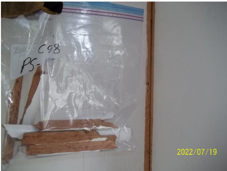
Photo 27: View of paint sample C98 PS-5, wall, outhouse interior.
