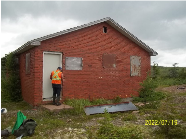
Photo 1: View of the accommodations cabin at Camp 98.
