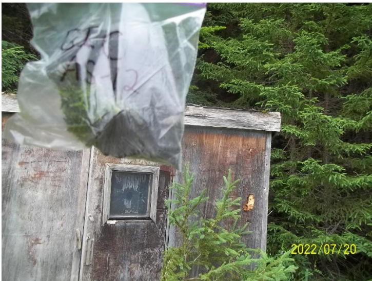
Photo 23: View of bulk material sample GIC AS-12, shingle, outhouse exterior.
