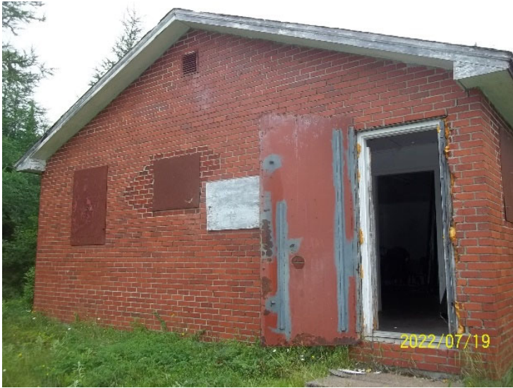
Photo 1: View of the accommodations cabin at Camp 50 site.
