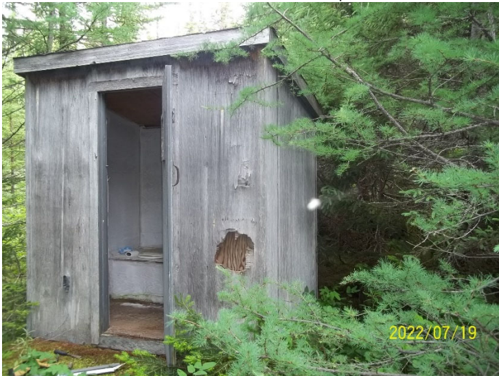
Photo 11: View of the outhouse at Camp 50 site.
