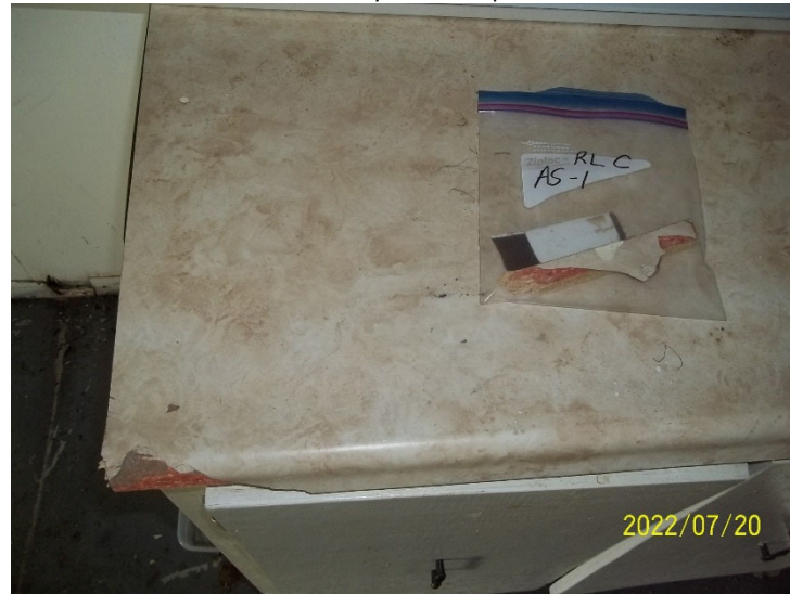
Photo 8: View of bulk material sample RLC AS-1, countertop mastic, cabin interior.
