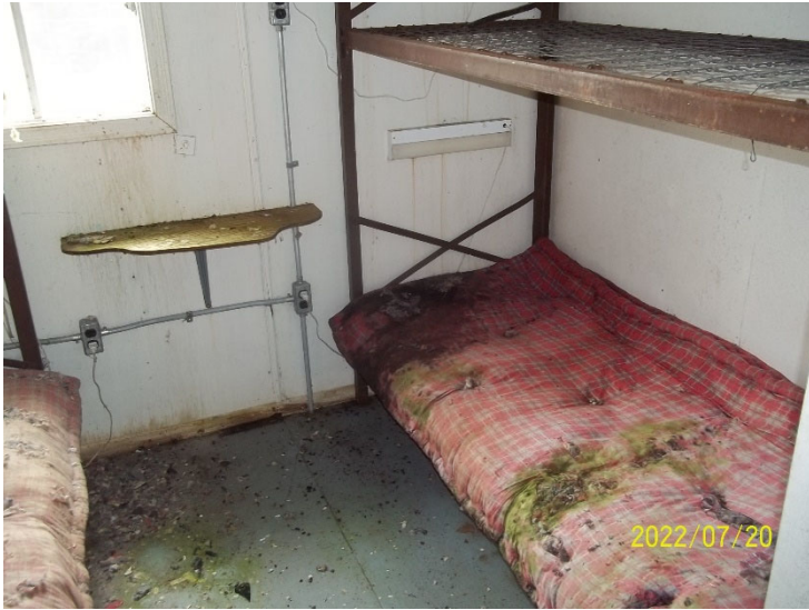
Photo 33: View of fluorescent light fixture in sleeping area of the accommodations cabin.
