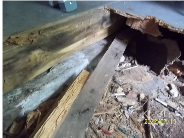
Photo 10: View of the crawl space beneath the accommodations cabin at Camp 50.
