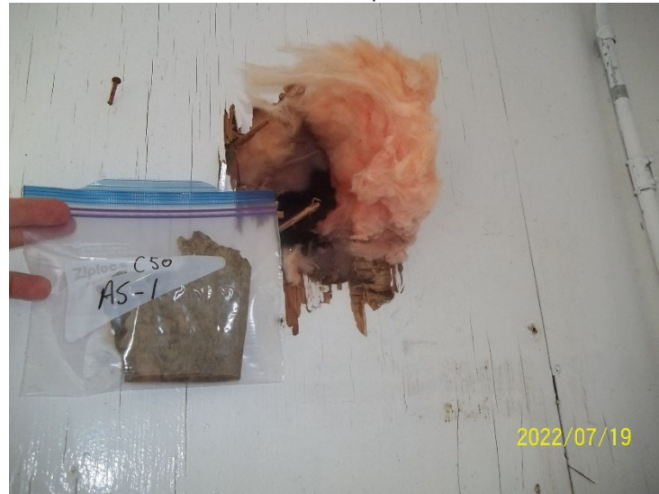
Photo 12: View of bulk material sample C50 AS-1, tar paper, cabin interior.
