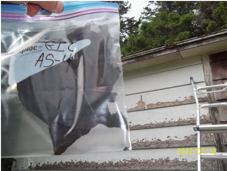
Photo 15: View of bulk material sample GIC AS-4, shingle, tar felt and tar paper, cabin exterior. 1.8% Chrysotile asbestos.
