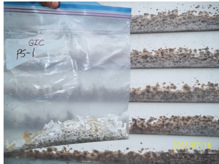
Photo 24: View of paint sample GIC PS-1, wall, cabin exterior.
