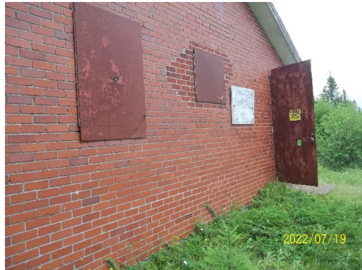
Photo 4: View of the accommodations cabin at Camp 50 site.
