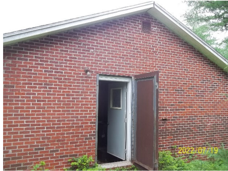
Photo 2: View of the accommodations cabin at Camp 50 site.
