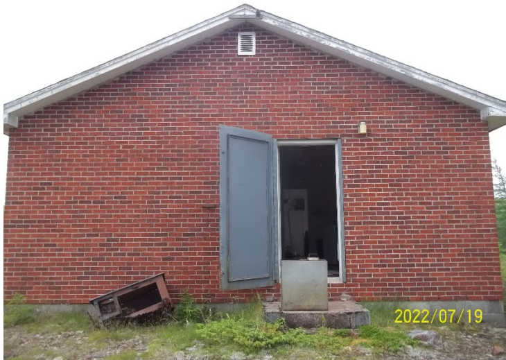
Photo 3: View of the accommodations cabin at Camp 98.
