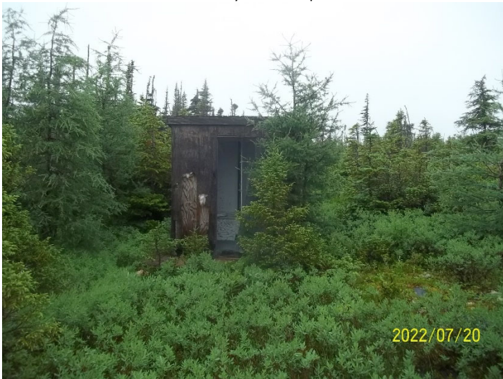
Photo 7: View of the outhouse at Rainy Lake Camp.
