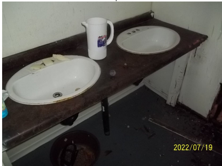
Photo 7: View of the washroom of the accommodations cabin at Camp 98.
