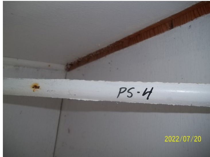
Photo 20: View of paint sample RLC PS-4, trim, outhouse interior.
