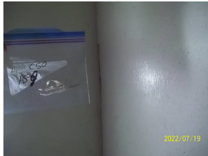
Photo 20: View of bulk material sample C50 AS-9, caulking, cabin interior.
