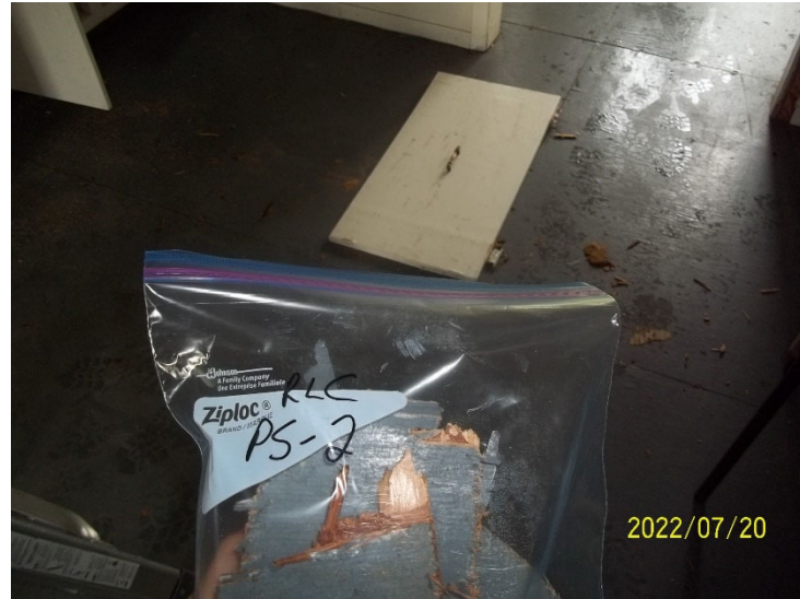
Photo 18: View of paint sample RLC PS-2, floor, cabin interior.
