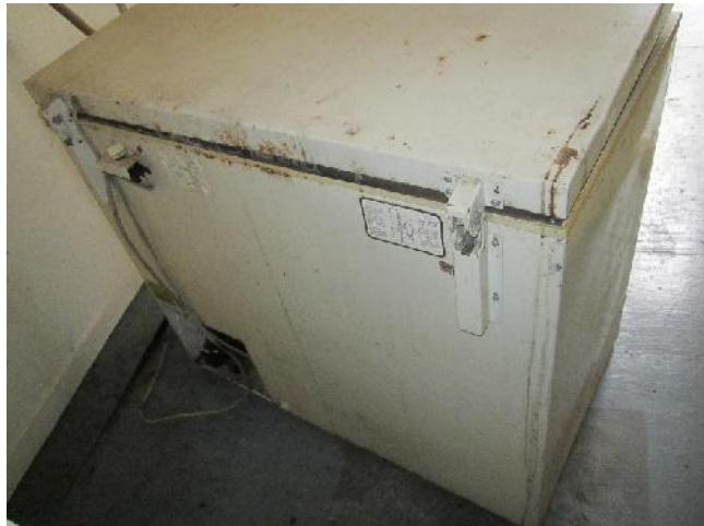
Photo 32: View of freezer, containing R12 reffridgerant, cabin interior.
