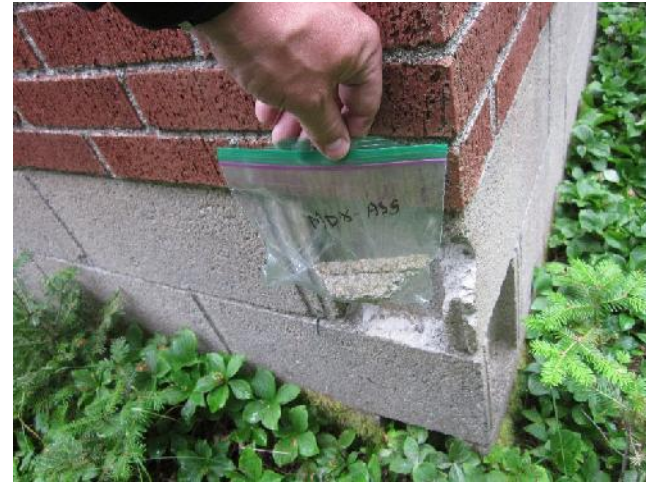
Photo 18: View of bulk material sample MDX-AS5, concrete block, cabin exterior.
