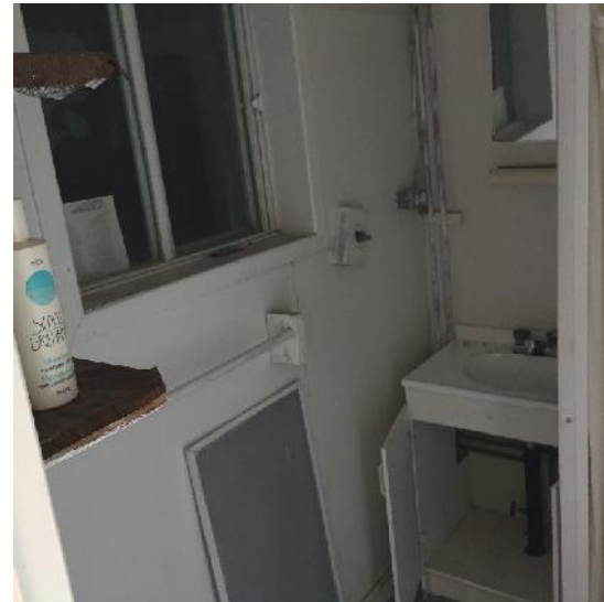
Photo 12: View of the bathroom in the accommodations cabin at Camp #2.
