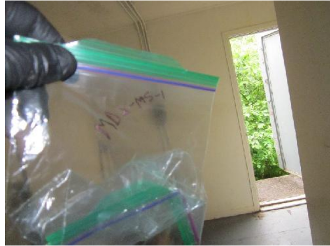
Photo 30: View of mould sample MDX-MS-1, cabin interior.
