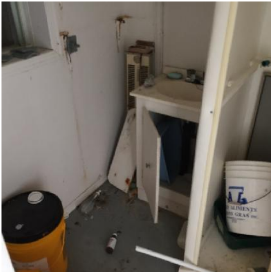
Photo 11: View of the washroom (Room 3) inside the accommodations cabin at Camp #1.
