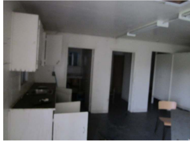
Photo 6: View of the kitchen/bunk area at Hungry Grove Pond Camp.
