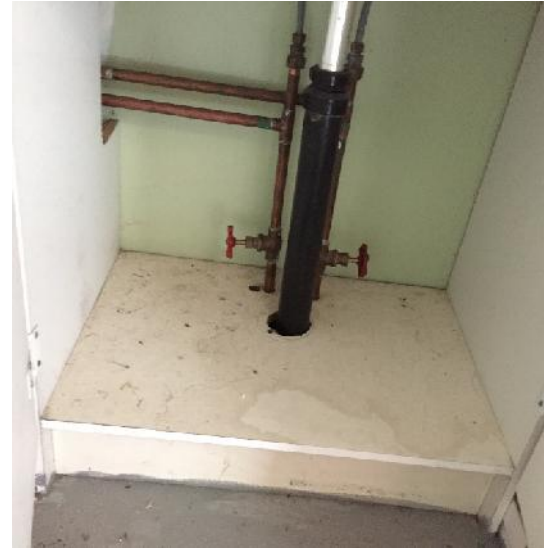
Photo 34: View of copper piping under bathroom sink, cabin interior.
