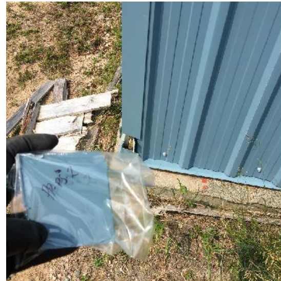
Photo 24: View of paint sample PP-PS2, wall, cabin exterior.
