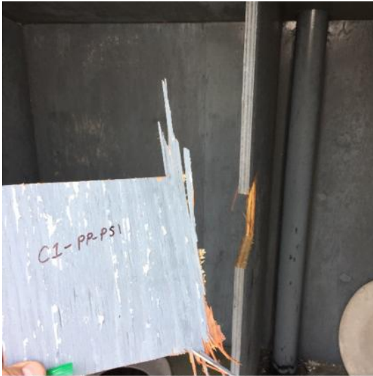
Photo 29: View of paint sample C1-PP-PS1, wall, outhouse interior.
