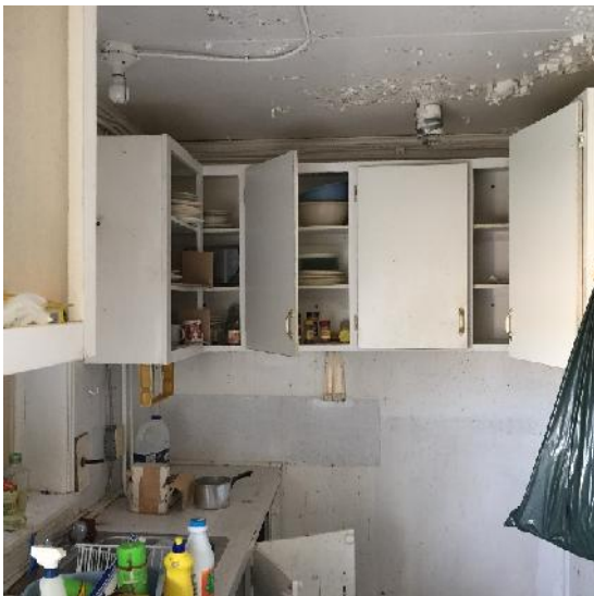
Photo 7: View of the kitchen (Room 1) inside the accommodations cabin at Camp #1.
