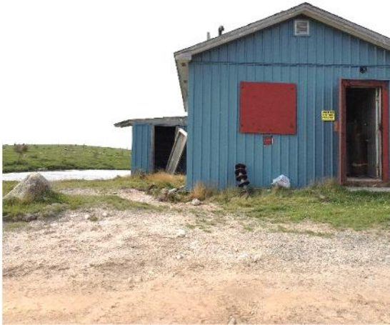
Photo 5: View of the accommodations cabin at Camp #1 site, looking northwest (Note: attached generator shed).
