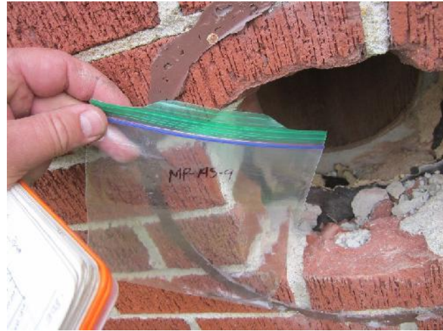
Photo 22: View of bulk material sample MP-AS9, red sealant, cabin exterior.
