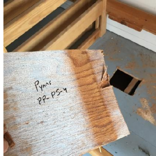
Photo 26: View of paint sample PP-PS4, ceiling, cabin interior.
