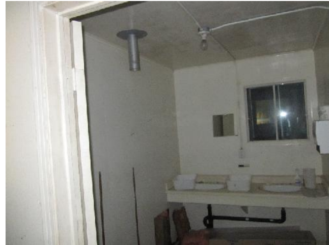
Photo 8: View of the bathroom at Medonnegonik Camp.
