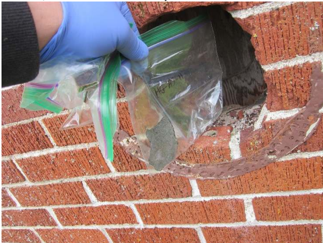
Photo 23: View of bulk material sample HG-AS11, tar paper, cabin exterior.
