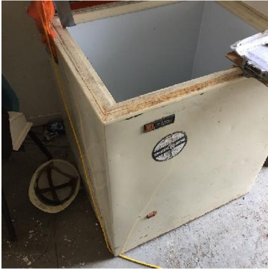
Photo 33: View of freezer inside the accomodations cabin, containing R12 refridgerant.
