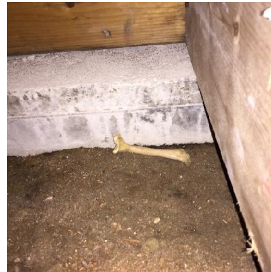
Photo 16: View of cavity inspection in the floor of cabin.
