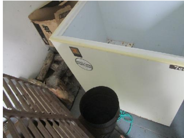
Photo 34: View of freezer, containing R12 reffridgerant, cabin interior.
