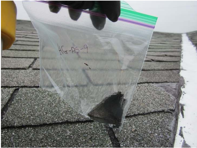
Photo 21: View of bulk material sample HG-AS9, black shingle and tar, cabin exterior. 4.8 % Crysofile Asbestos.
