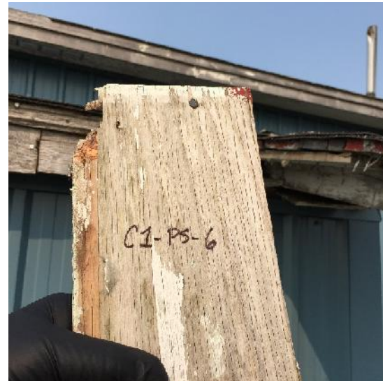
Photo 28: View of paint sample C1-PS6, wall, cabin exterior.
