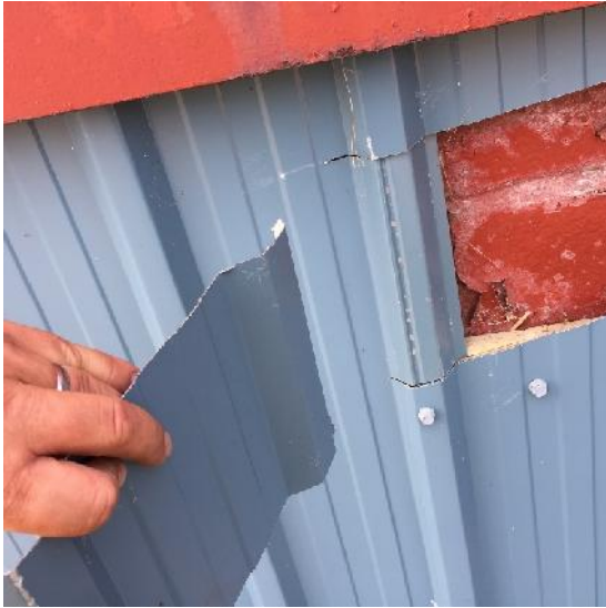
Photo 25: View of paint sample C1-PS3, wall, cabin exterior.
