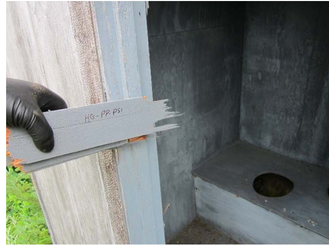
Photo 30: View of paint sample HG-PS1, grey, outhouse interior.
