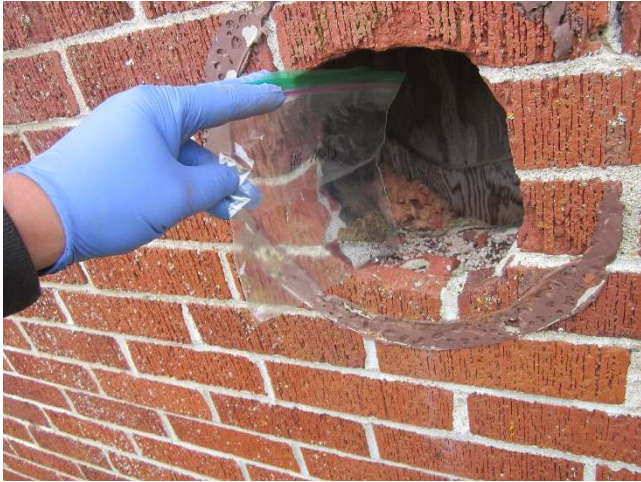
Photo 25: View of bulk material sample HG-AS-13, tar paper, cabin exterior.
