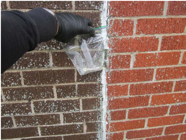
Photo 15: View of bulk material sample HG-AS3, white caulking, cabin exterior.
