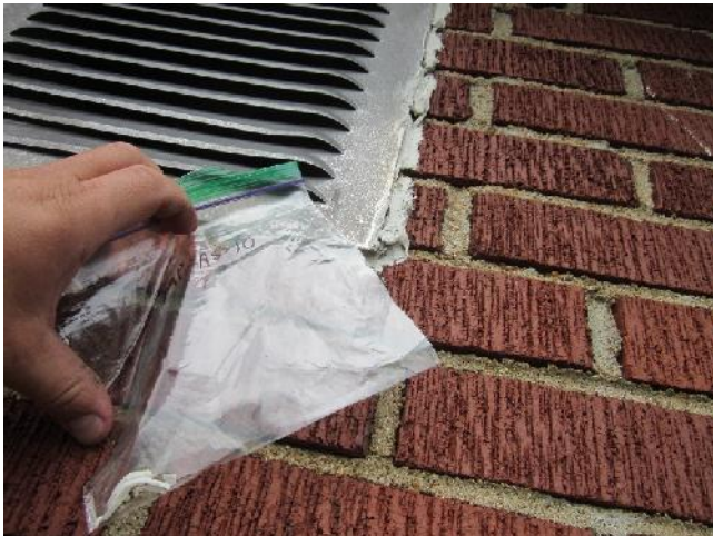
Photo 23: View of bulk material sample MP-AS10, white caulking, cabin exterior.
