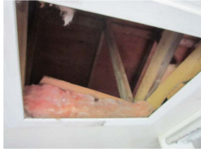
Photo 10: View of attic in accommodations cabin at Hungry Grove Pond Camp.
