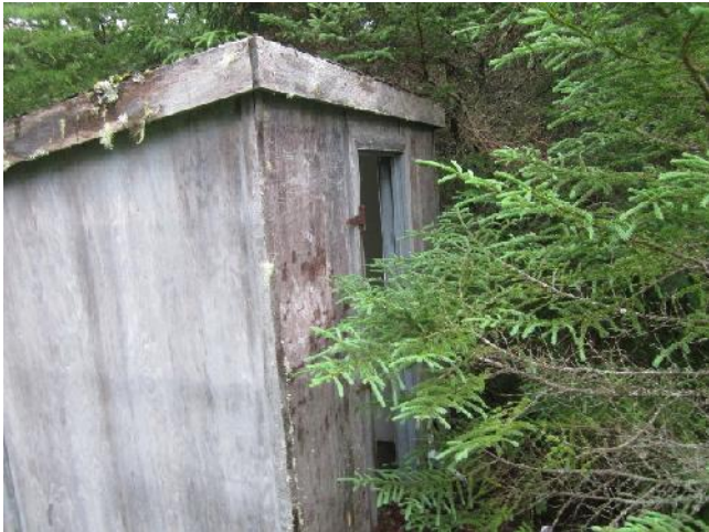
Photo 11: View of the exterior of the outhouse at Camp 100.
