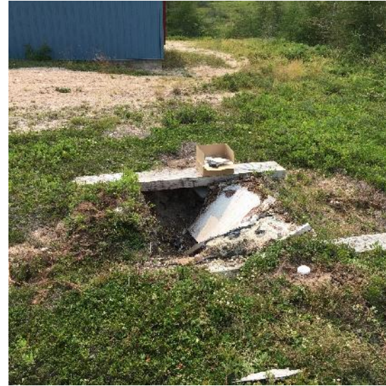
Photo 14: View of outhouse foundation, looking southwest.
