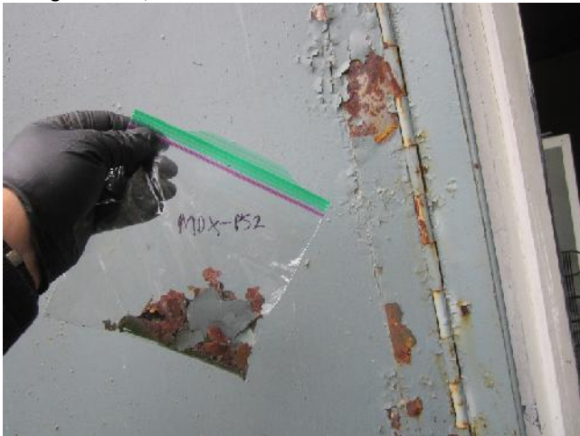
Photo 27: View of paint sample MDX-PS2, grey, cabin exterior.
