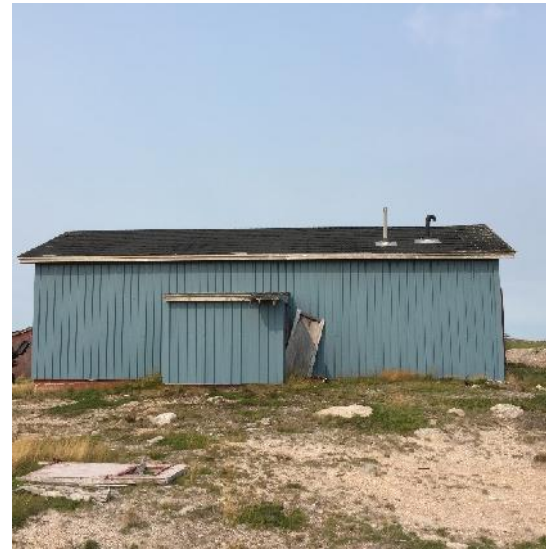
Photo 6: View of the accommodations cabin at Camp #1 site, looking northeast (Note: attached generator shed).
