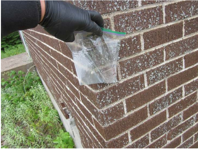
Photo 13: View of bulk material sample HG-AS1, brown brick, cabin exterior.
