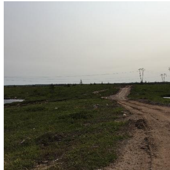
Photo 4: View of the gravel access road at Camp #1 site, looking southwest.
