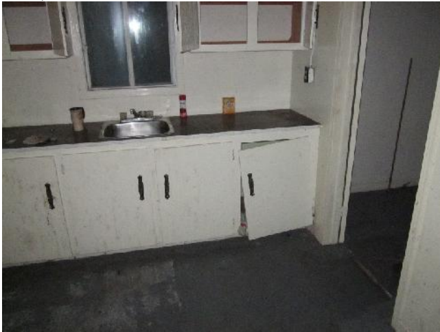
Photo 7: View of the kitchen area at Medonnegonik Camp.
