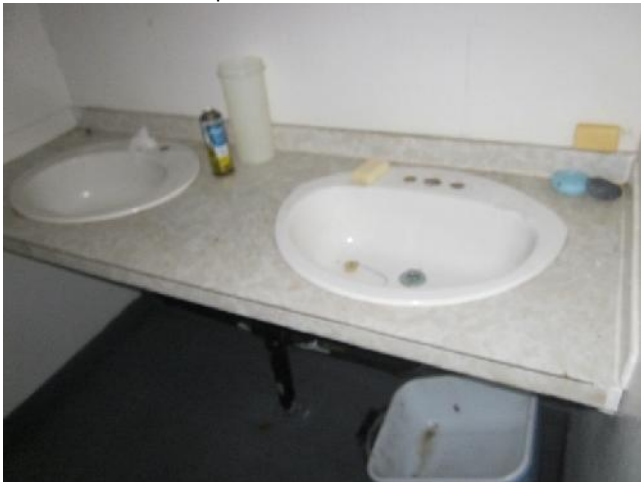
Photo 7: View of the bathroom at Mitchell's Pond Camp.
