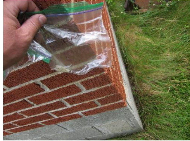
Photo 18: View of bulk material sample MP-AS5, grey mortar, cabin exterior.
