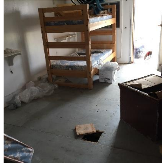
Photo 10: View of the bedroom (Room 2) inside the accommodations cabin at Camp #1.
