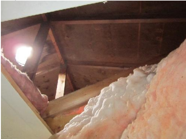
Photo 11: View of attic of accommodations cabin at Mitchell's Pond Camp.
