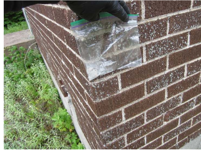
Photo 14: View of bulk material sample HG-AS2, grey mortar, cabin exterior.
