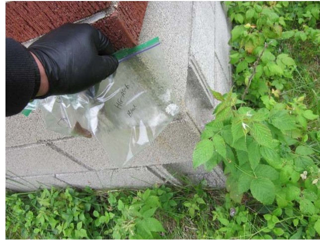
Photo 18: View of bulk material sample HG-AS6, concrete block, cabin exterior.
