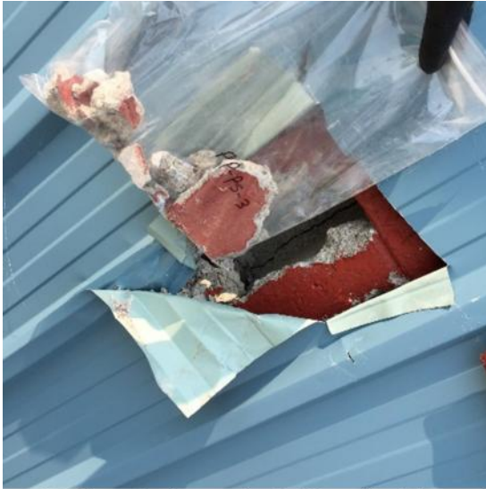
Photo 25: View of paint sample PP-PS3, wall, cabin exterior.
