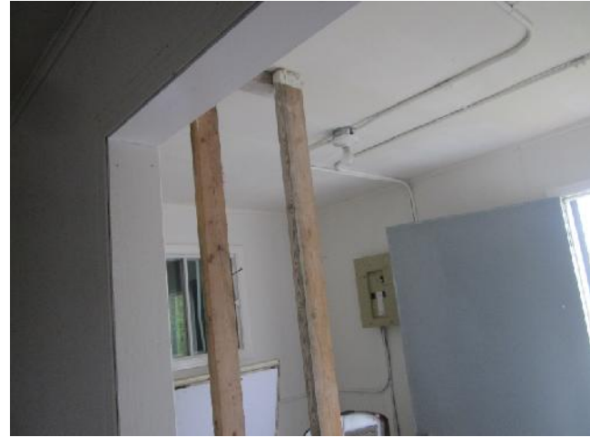
Photo 6: View of the pantry area at Mitchell's Pond Camp.
