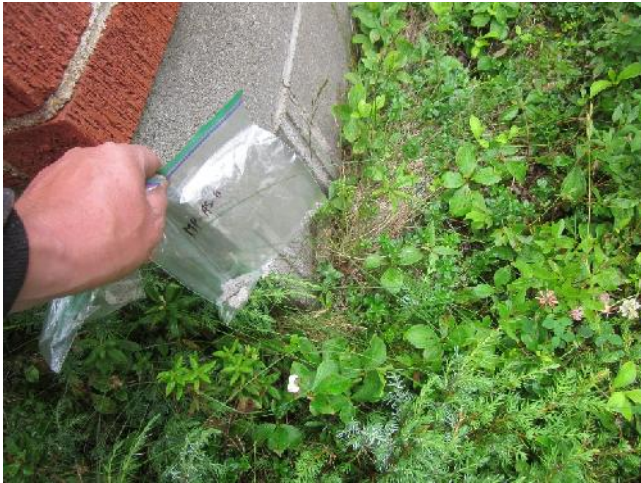
Photo 19: View of bulk material sample MP-AS6, grey mortar, cabin exterior.
