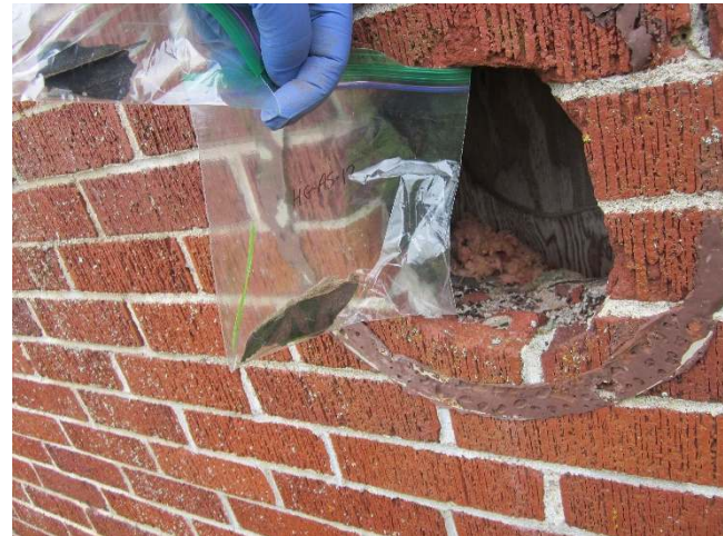
Photo 24: View of bulk material sample HG-AS12, pressed board, cabin exterior.
