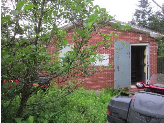
Photo 1: View of the accommodations cabin at Medonnegonik Camp, looking south.
