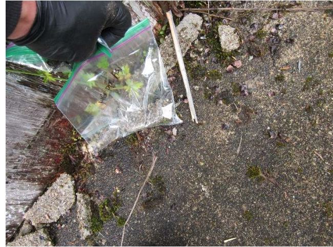
Photo 26: View of bulk material sample HG-PP-AS1, concrete, outhouse exterior.
