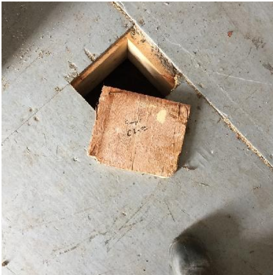
Photo 23: View of paint sample C1-PS1, floor, cabin interior.
