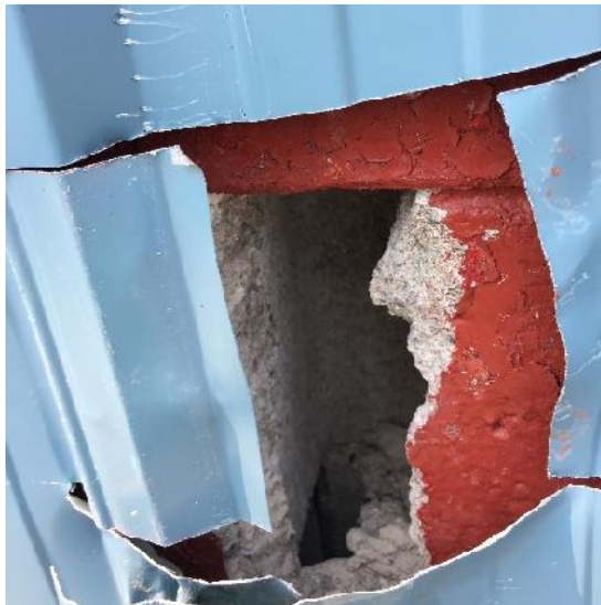
Photo 15: View of cavity inspection on the exterior of cabin.
