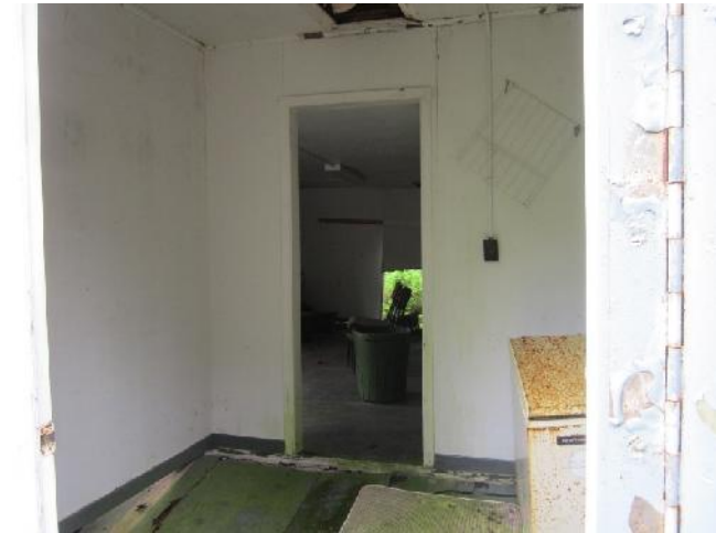
Photo 8: View of the pantry area in the accommodations cabin at Camp 100.
