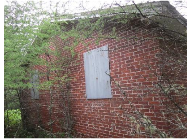
Photo 4: View of the accommodations cabin at Camp 100, looking east.
