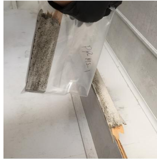
Photo 30: View of bulk mould sample PP-MS1, wall of cabin interior.
