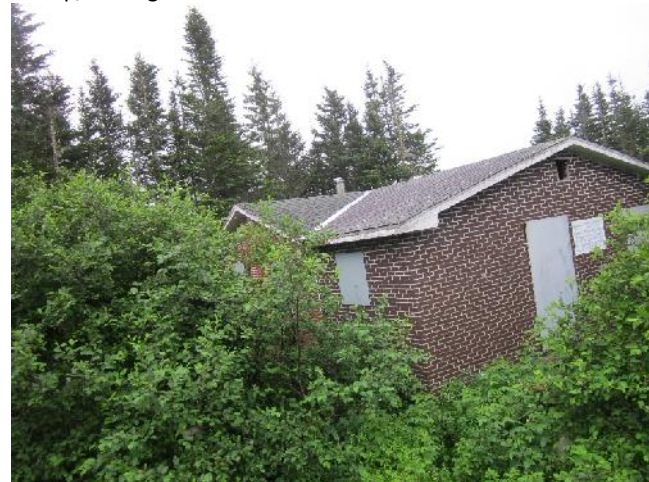
Photo 4: View of the accommodations cabin at Medonnegonik Camp, looking northwest.
