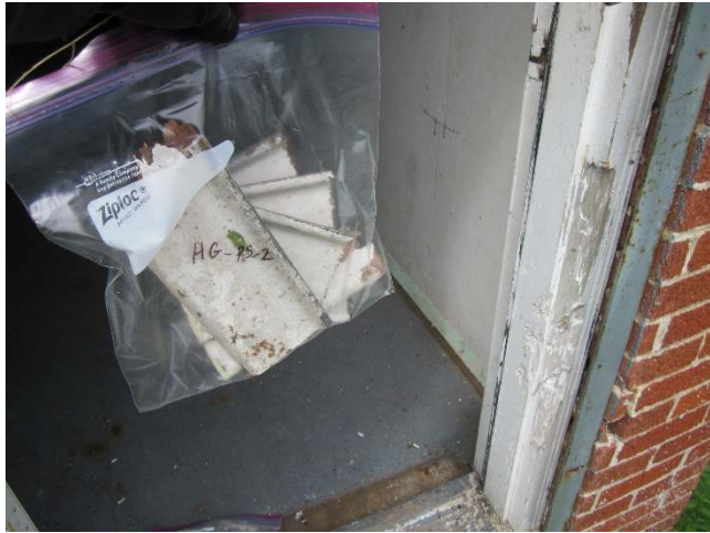
Photo 29: View of paint sample HG-PS2, grey, accommodations cabin interior.
