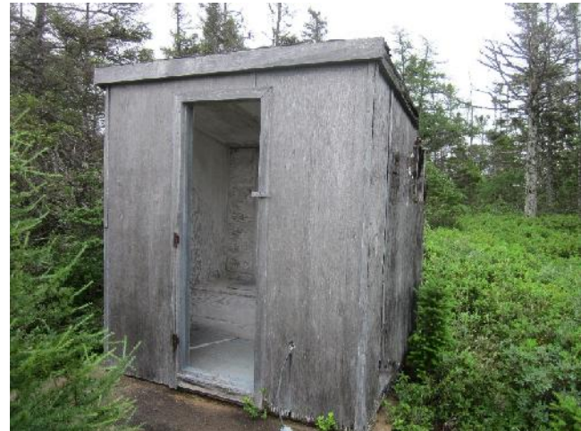
Photo 8: View of the outhouse at Mitchell's Pond Camp.
