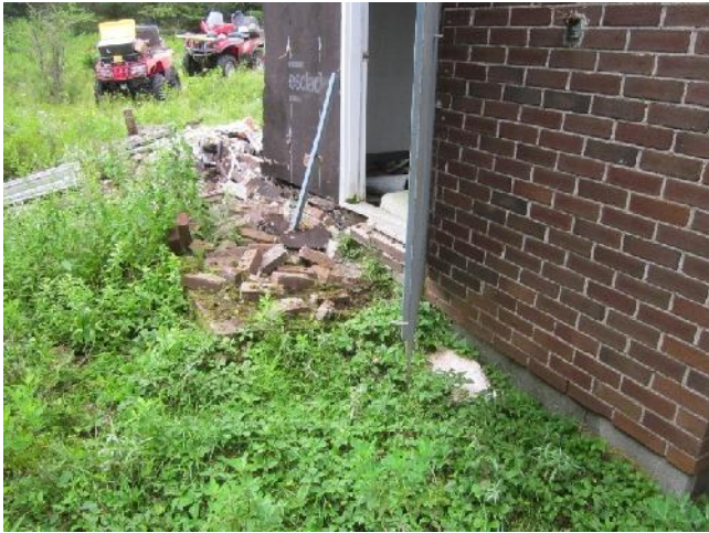
Photo 5: View of the accommodations cabin at Camp 100, looking east.
