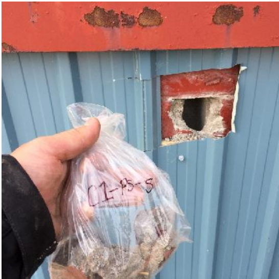
Photo 27: View of paint sample C1-PS5, wall, cabin exterior.
