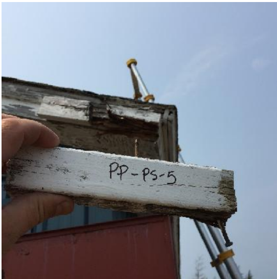
Photo 27: View of paint sample PP-PS5, wall, cabin exterior.
