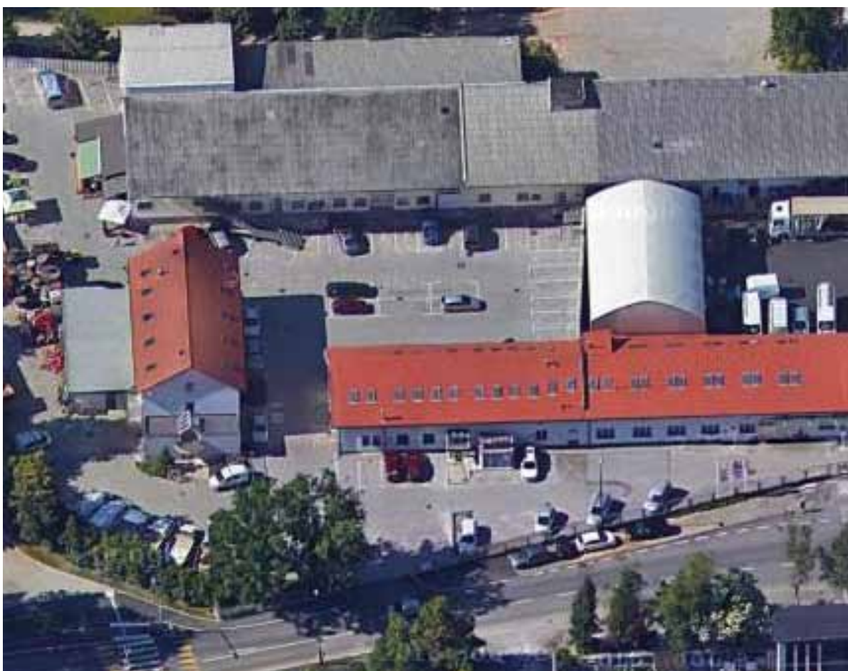
OMEGA AIR production plant in Ljubljana, Slovenia
