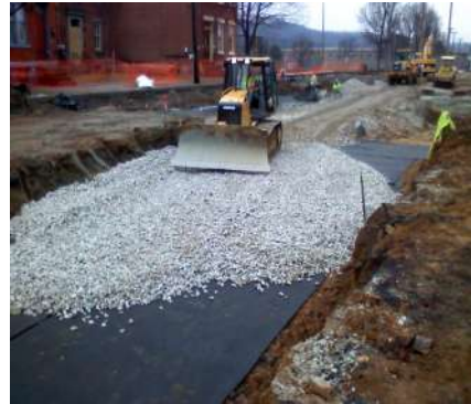
Installation of Foundation Mat and Base Course
