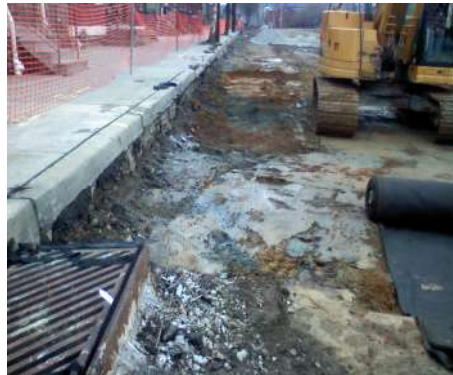
Overexcavation of Unsuitable Material
