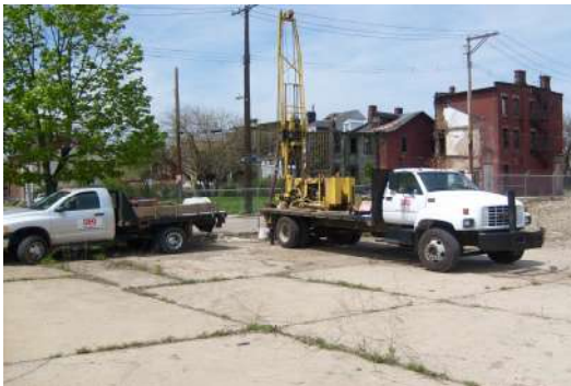
Drill Rig on Project Site
