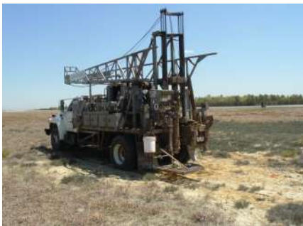
Drill Rig on Project Site
