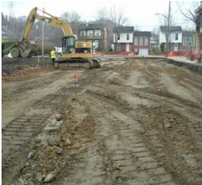
Test Pit Investigation
