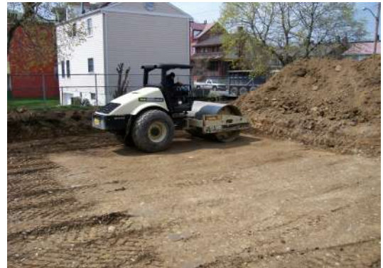
Site Preparation Activity
