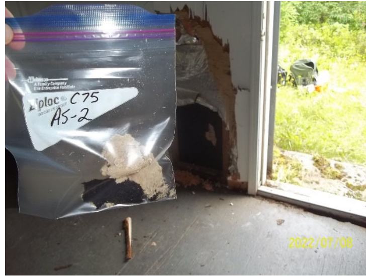
Photo 14: View of bulk material sample C75 AS-2, particle board, cabin interior.
