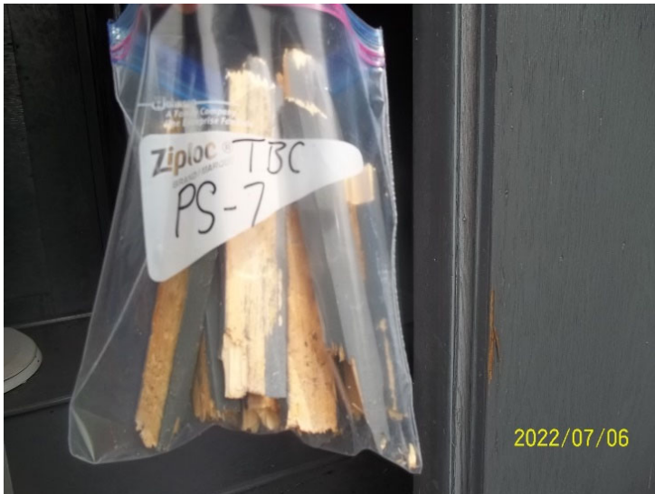
Photo 27: View of paint sample TBC PS-7, door, outhouse interior.
