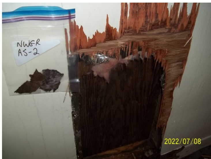
Photo 13: View of bulk material sample NWGR AS-2, tar paper, cabin interior.
