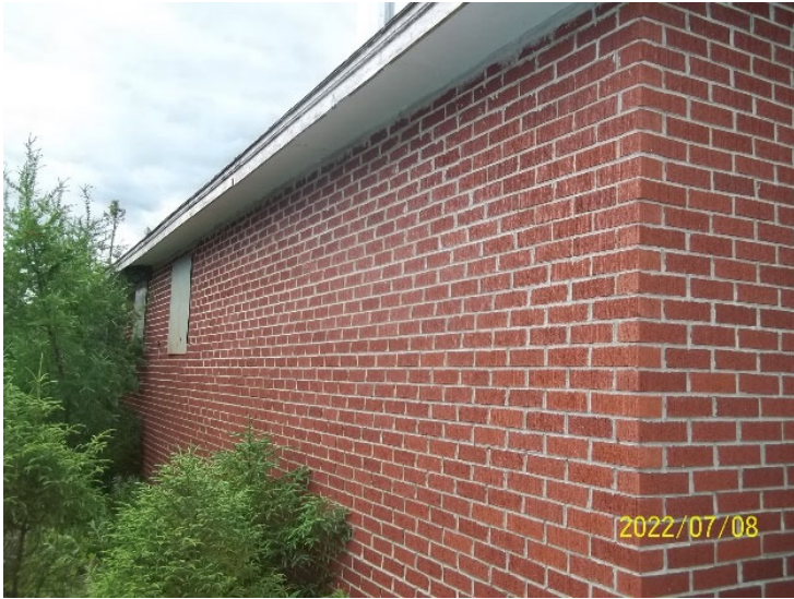
Photo 1: View of the accommodations cabin at Camp 75 site.
