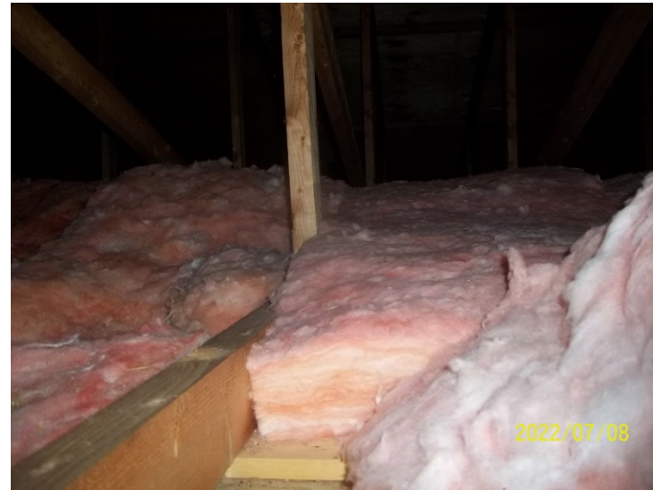
Photo 12: View of the attic in the accommodations cabin at Camp 130.
