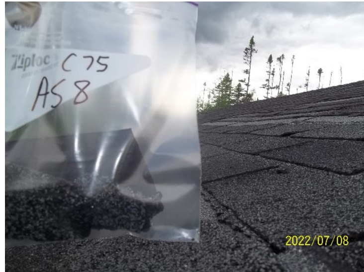
Photo 20: View of bulk material sample C75 AS-8, shingle, cabin exterior.
