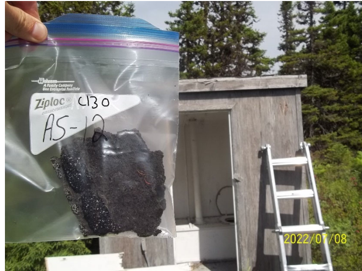
Photo 26: View of bulk material sample C130 AS-12, shingle, outhouse exterior.
