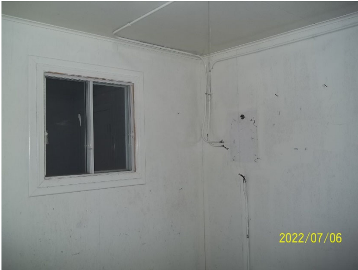
Photo 21: View of former location of electrical panel, cabin interior.
