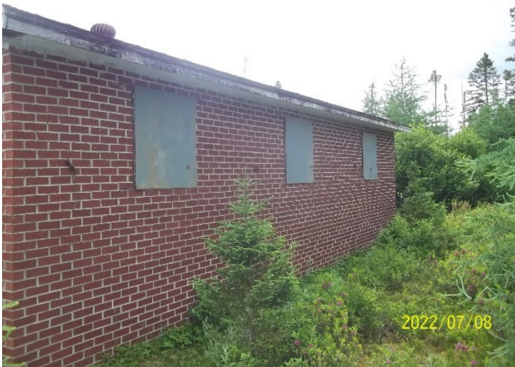
Photo 3: View of the accommodations cabin at Camp 75 site.
