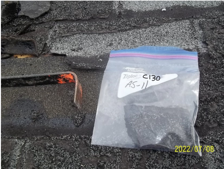
Photo 25: View of bulk material sample C130 AS-11, shingle, cabin exterior.
