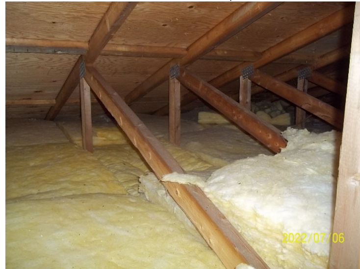
Photo 8: View of attic in accommodations cabin at Pot Hill Camp.
