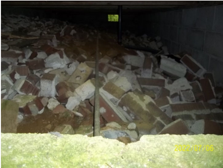
Photo 9: View of crawl space beneath accommodations cabin at Pot Hill Camp.
