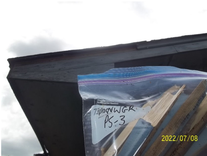
Photo 23: View of paint sample NWGR PS-3, roof, cabin exterior .
