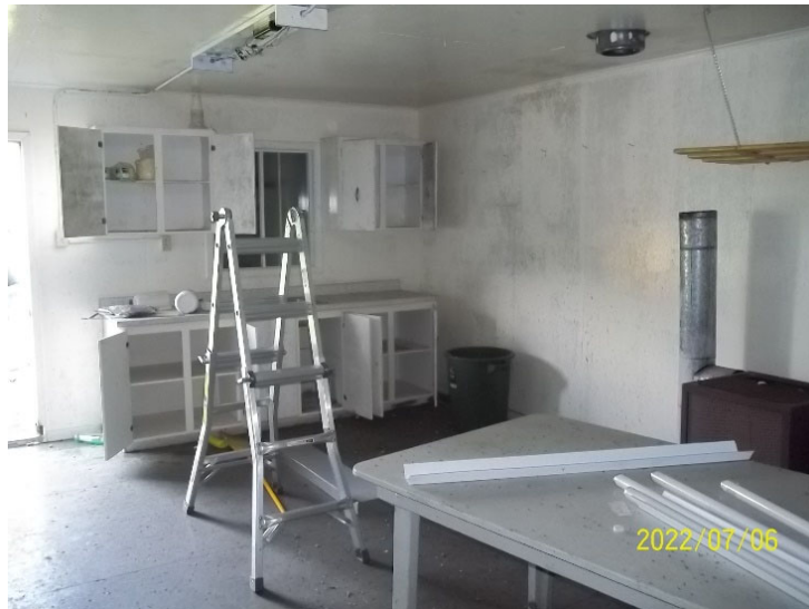
Photo 7: View of the kitchen area of the accommodations cabin at Three Brooks Camp.
