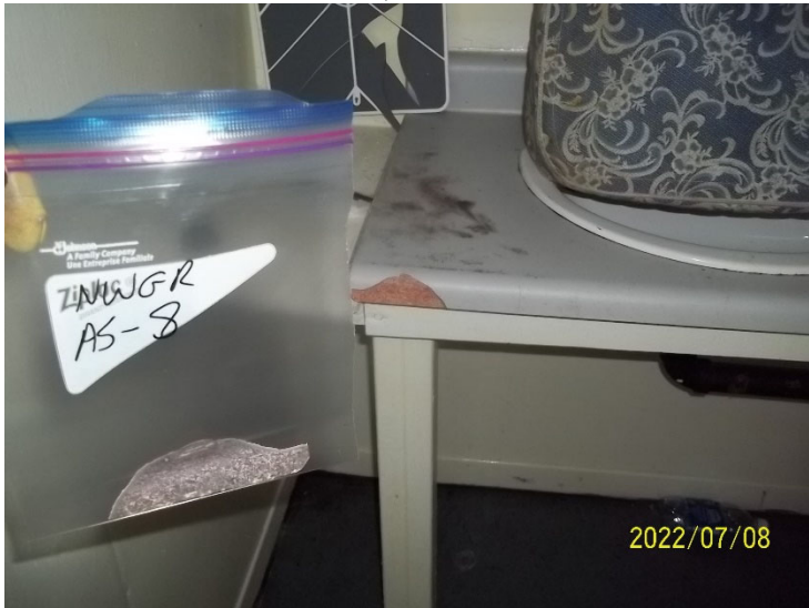
Photo 19: View of bulk material sample NWGR AS-8, countertop mastic, cabin interior.
