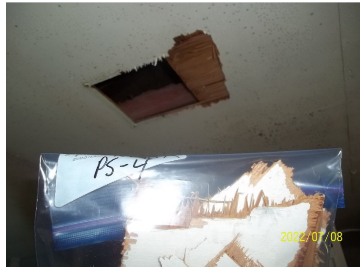
Photo 24: View of paint sample NWGR PS-4, ceiling, cabin interior.
