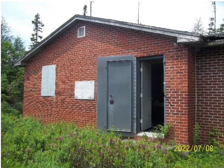
Photo 7: View of accomodations cabin at North West Gander River Camp.
