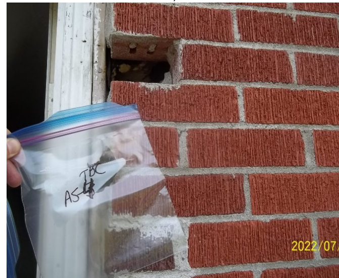
Photo 16: View of bulk material sample TBC AS-4, tar paper, cabin exterior.
