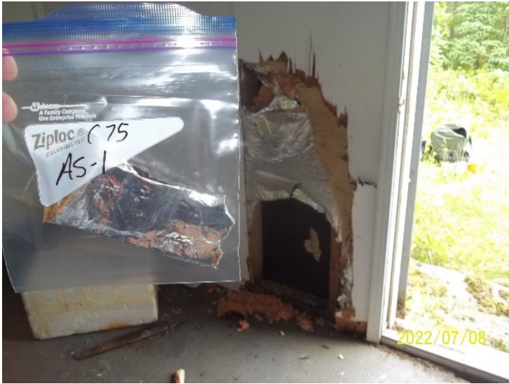
Photo 13: View of bulk material sample C75 AS-1, foil paper, cabin interior.
