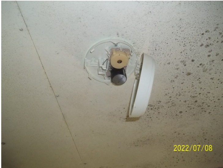
Photo 33: View of smoke detector inside the accommodations cabin.
