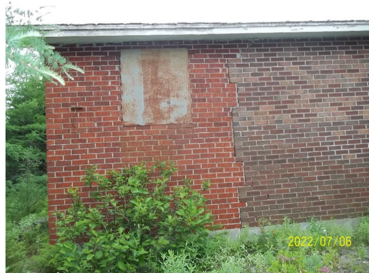
Photo 4: View of the accommodations cabin at Pot Hill Camp.
