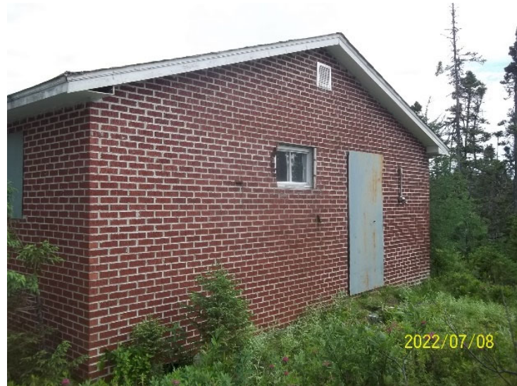
Photo 4: View of the accommodations cabin at Camp 75 site.
