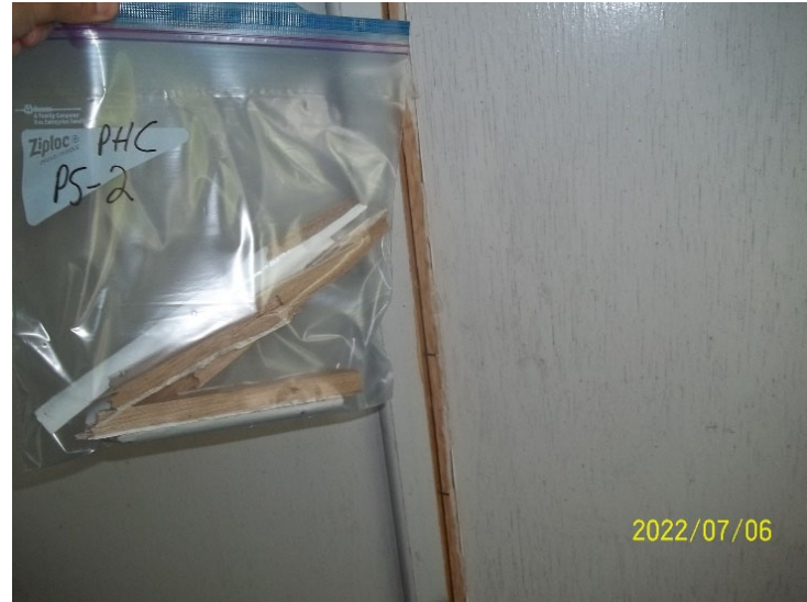
Photo 18: View of paint sample PHC PS-2, wall, cabin interior.
