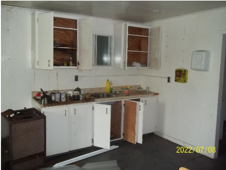
Photo 5: View of the kitchen area inside the accommodations cabin at Camp 75.
