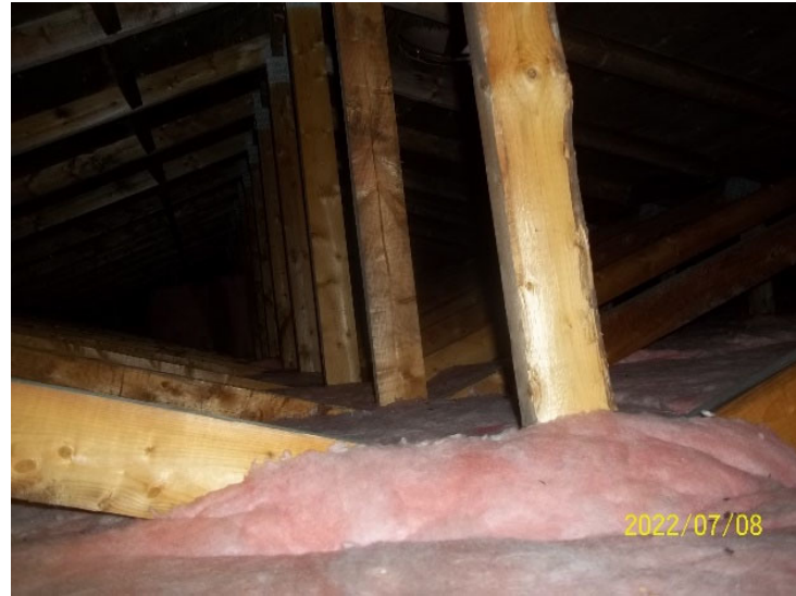
Photo 10: View of the attic inside the accommodations cabin at Camp 75.
