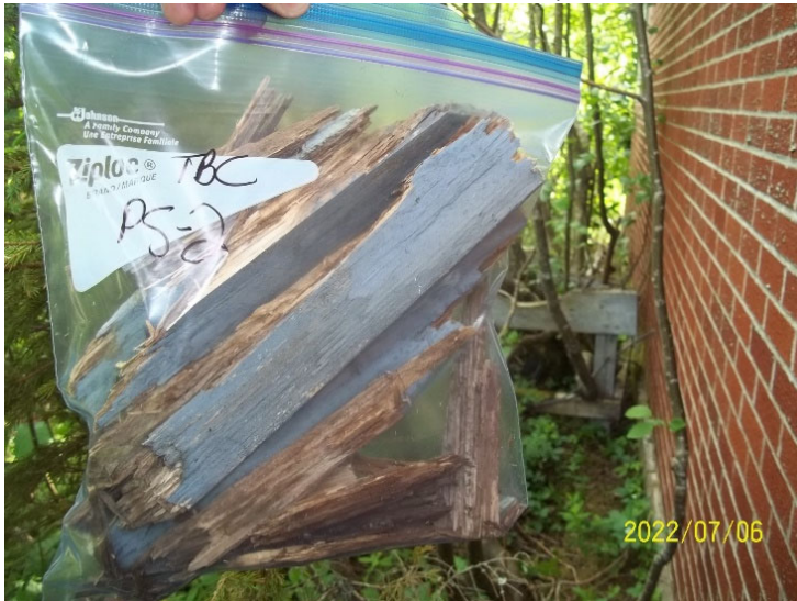
Photo 23: View of paint sample TBC PS-2, wood cradle, cabin exterior.
