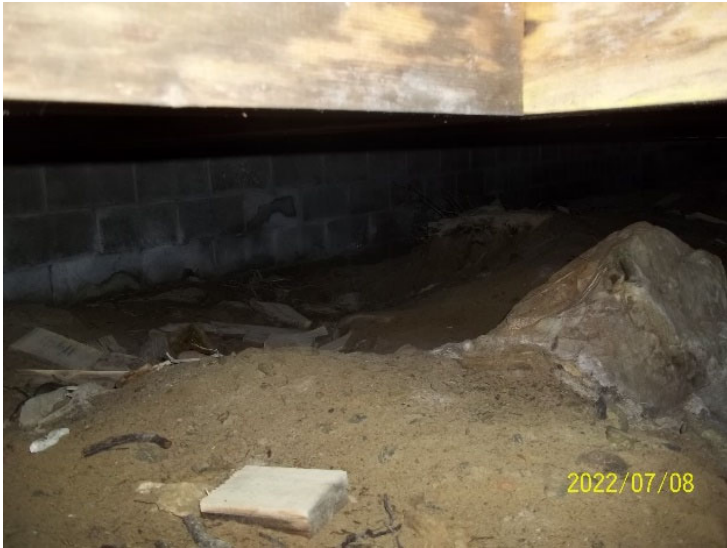
Photo 9: View of the crawl space beneath the accommodations cabin at Camp 75.
