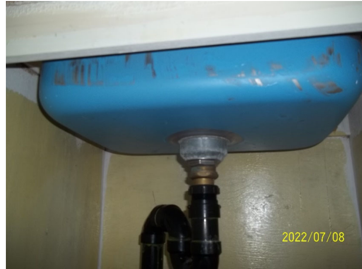
Photo 30: View of sink undercoating, cabin interior.
