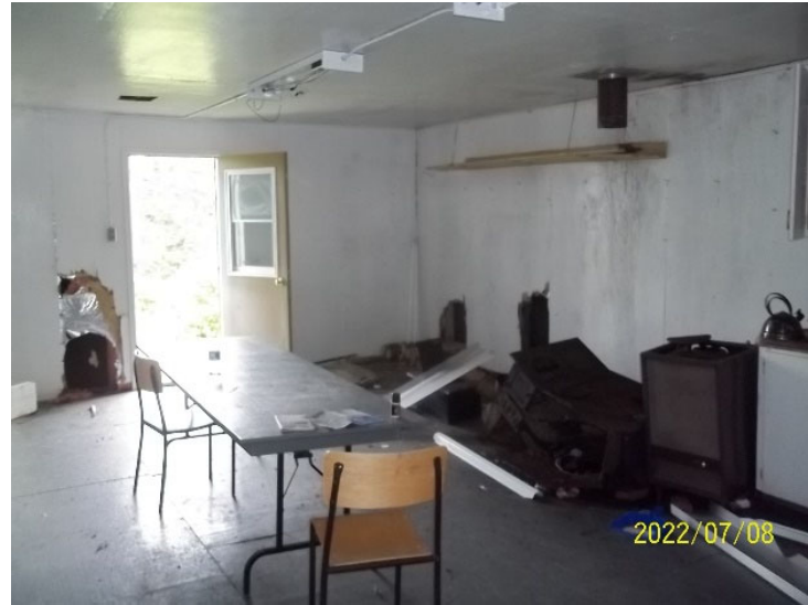
Photo 6: View of the dining area inside the accommodations cabin at Camp 75.
