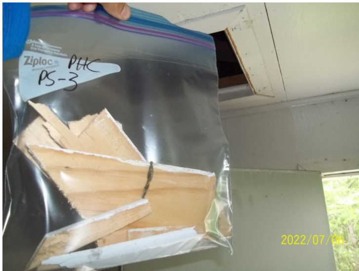
Photo 19: View of paint sample PHC PS-3, ceiling, cabin interior.
