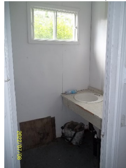
Photo 8: View of the washroom inside the accommodations cabin at Camp 75.
