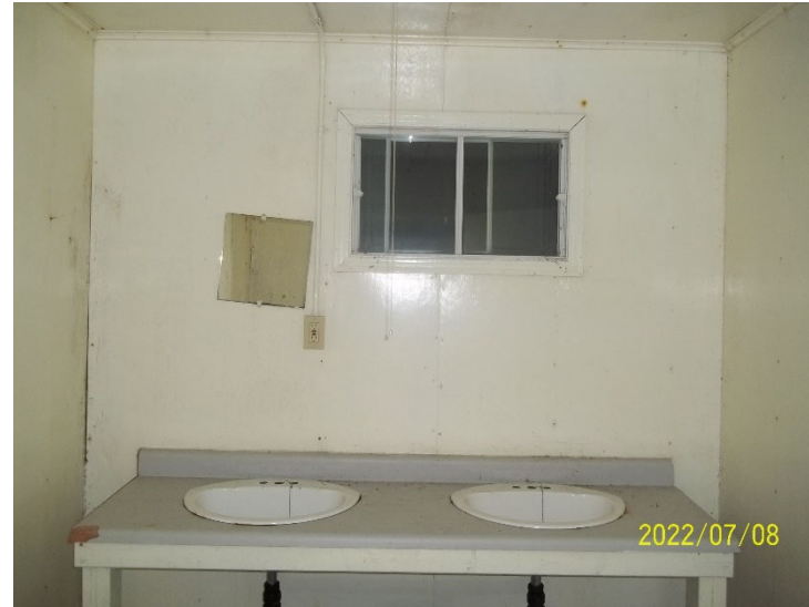
Photo 10: View of the washroom area of the accommodations cabin at Camp 130.
