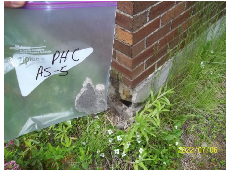
Photo 14: View of bulk material sample PHC AS-5, cinder block, cabin exterior.
