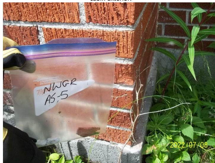
Photo 16: View of bulk material sample NWGR AS-5, brick and mortar, cabin exterior.
