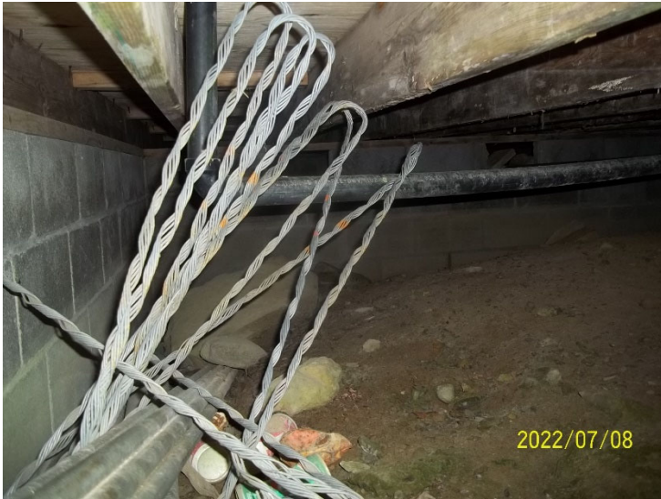
Photo 13: View of the crawl space beneath the accommodations cabin at Camp 130.
