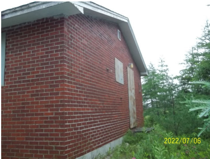
Photo 3: View of the accommodations cabin at Pot Hill Camp.
