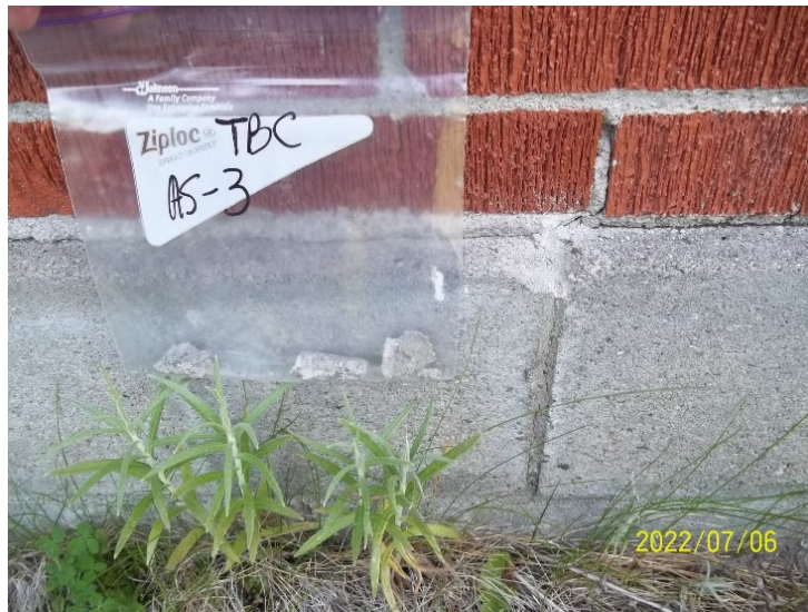
Photo 15: View of bulk material sample TBC AS-3, cinder block, cabin exterior.
