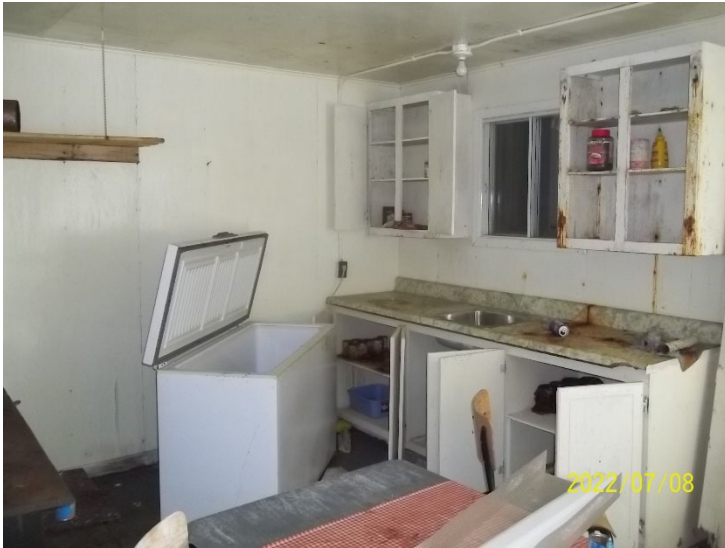
Photo 9: View of the kitchen area of the accommodations cabin at Camp 130.
