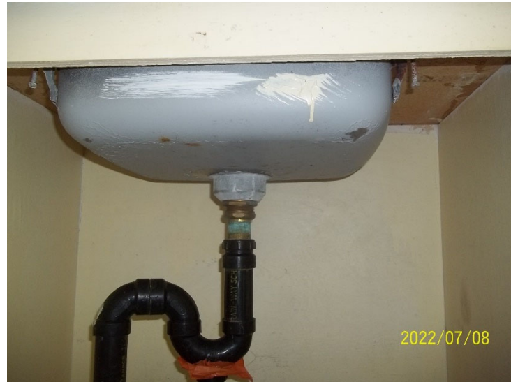
Photo 32: View of sink undercoating, cabin interior.
