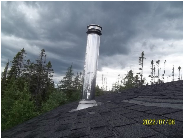
Photo 11: View of the roof on the accommodations cabin at Camp 75.
