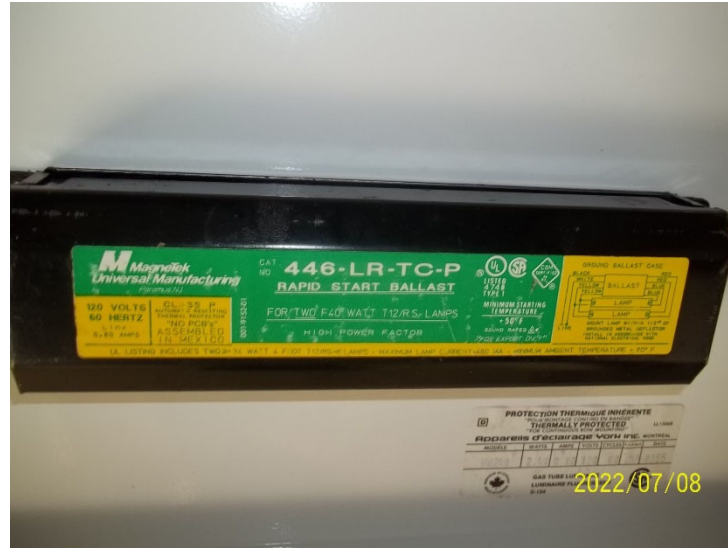
Photo 34: View of fluorescent light ballast. Note: label indicating no PCBs.
