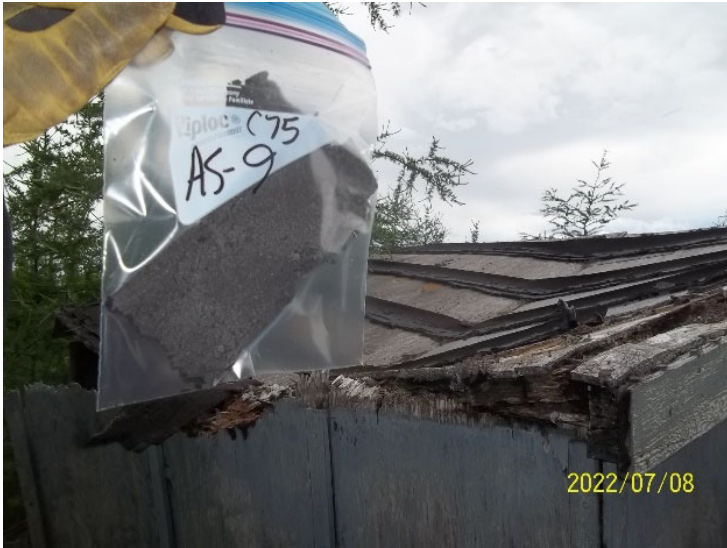
Photo 21: View of bulk material sample C75 AS-9, shingle, outhouse exterior.
