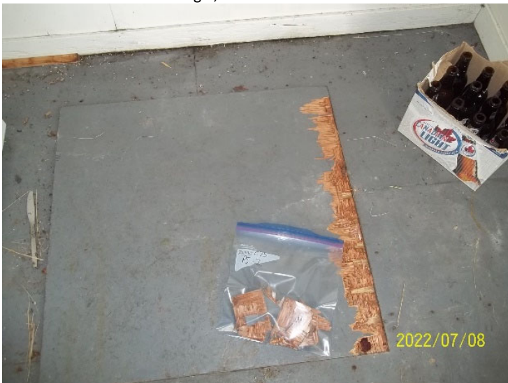
Photo 23: View of paint sample C75 PS-2, floor, cabin interior.
