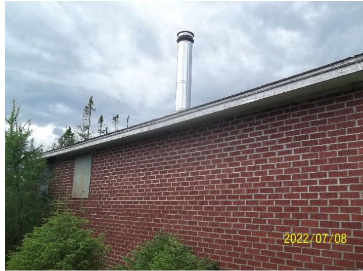
Photo 2: View of the accommodations cabin at Camp 75 site.
