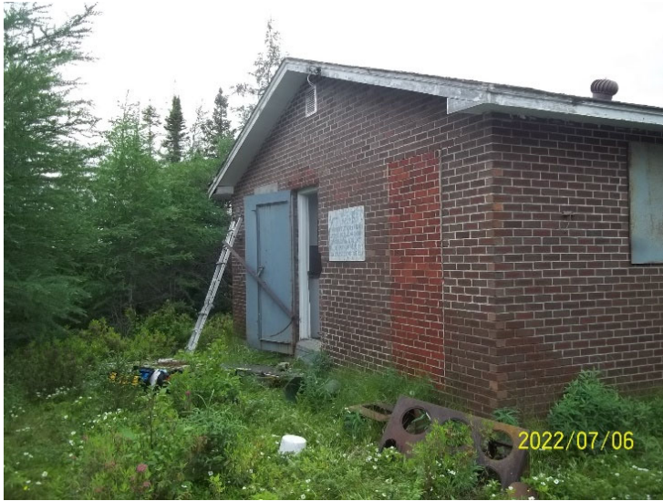
Photo 1: View of the accommodations cabin at Pot Hill Camp.
