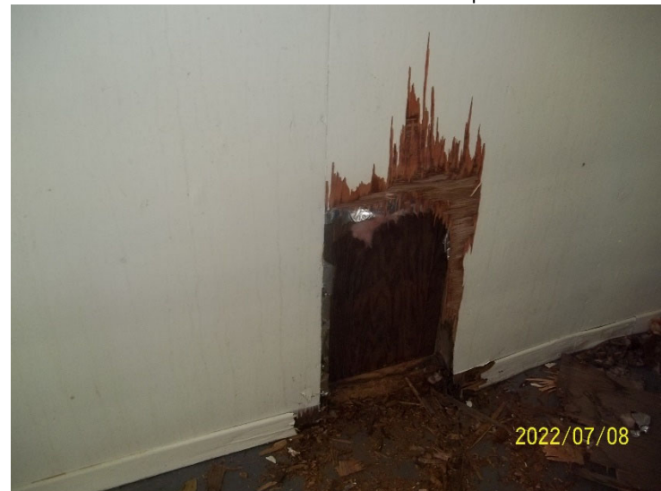
Photo 12: View of location of bulk material sample NWGR AS-1, foil paper, cabin interior .
