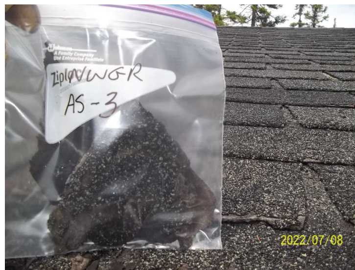
Photo 14: View of bulk material sample NWGR AS-3, shingle, cabin exterior.
