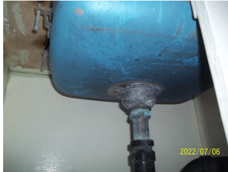
Photo 22: View of sink undercoating, cabin interior.
